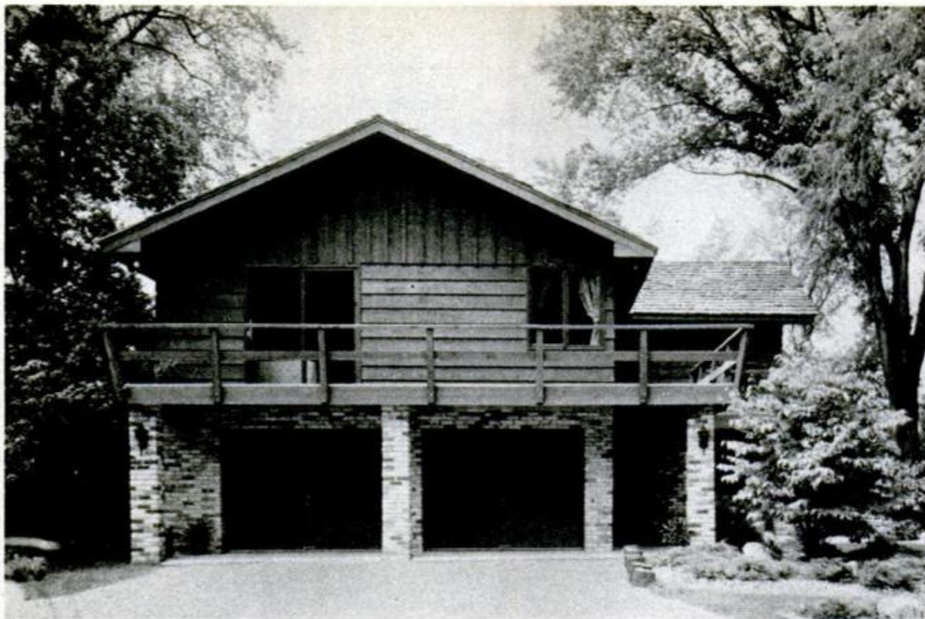
STREET SIDE OF HOUSE has pillars added, is now considered rear of house. Family room overlooks lake
