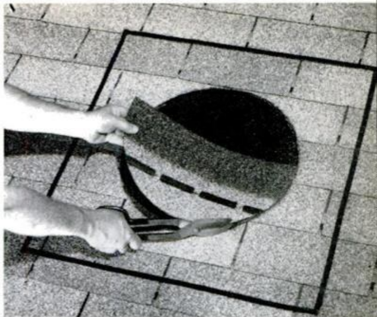
4. CUT HOLE THROUGH SHINGLES only with tin shears, then clear the shingles from inside the circle
