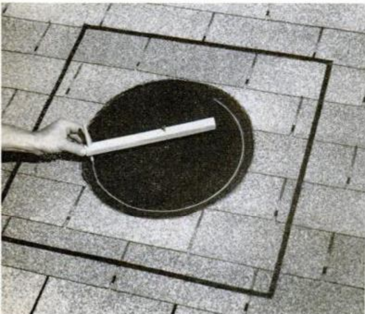
5. DRAW SECOND CIRCLE 15 in. in diameter with the compass on roofing paper inside the cleared area
