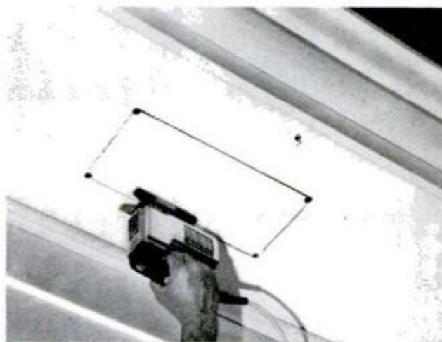
4. CUT HOLE THROUGH SHINGLES only with tin shears, then clear the shingles from inside the circle
