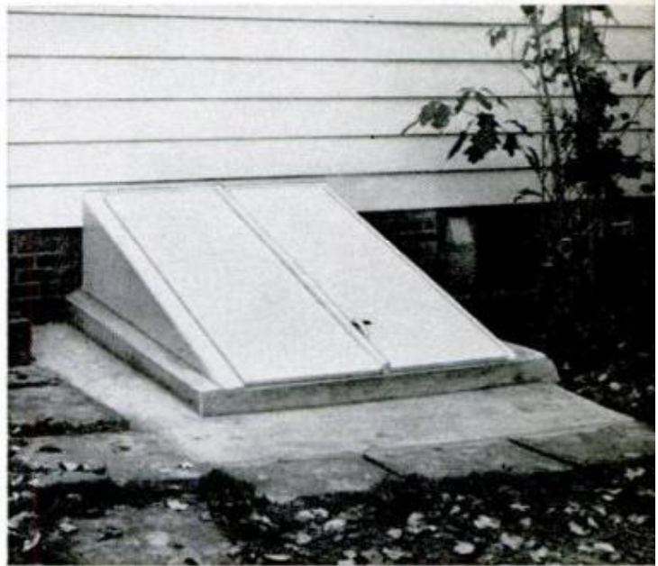
PITCHED CONCRETE LEDGE gives positive water runoff and makes lawn edge trimming a lot easier
