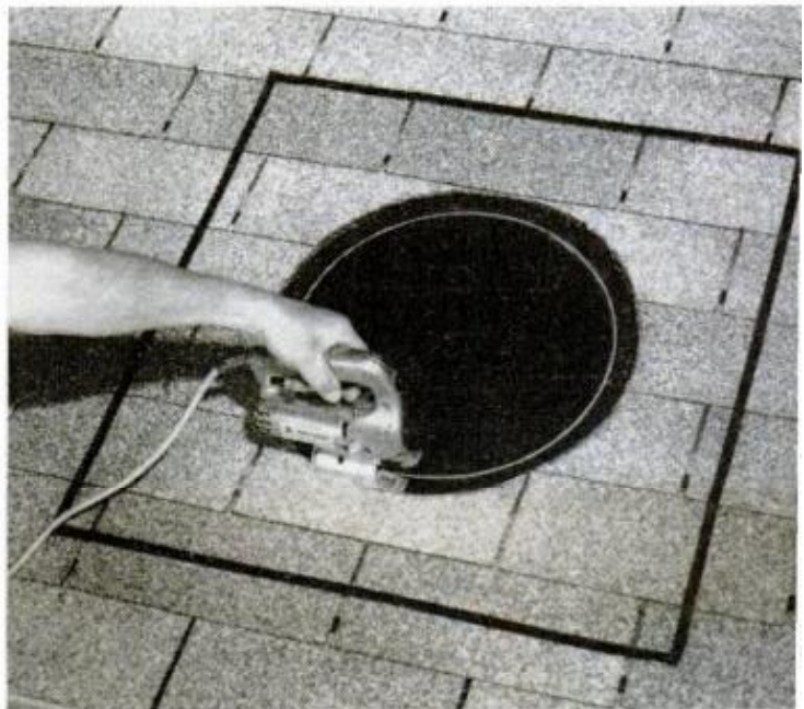
6. SAW THROUGH ROOF following the 15-in. circle, then slide flange of fan housing up under shingles
