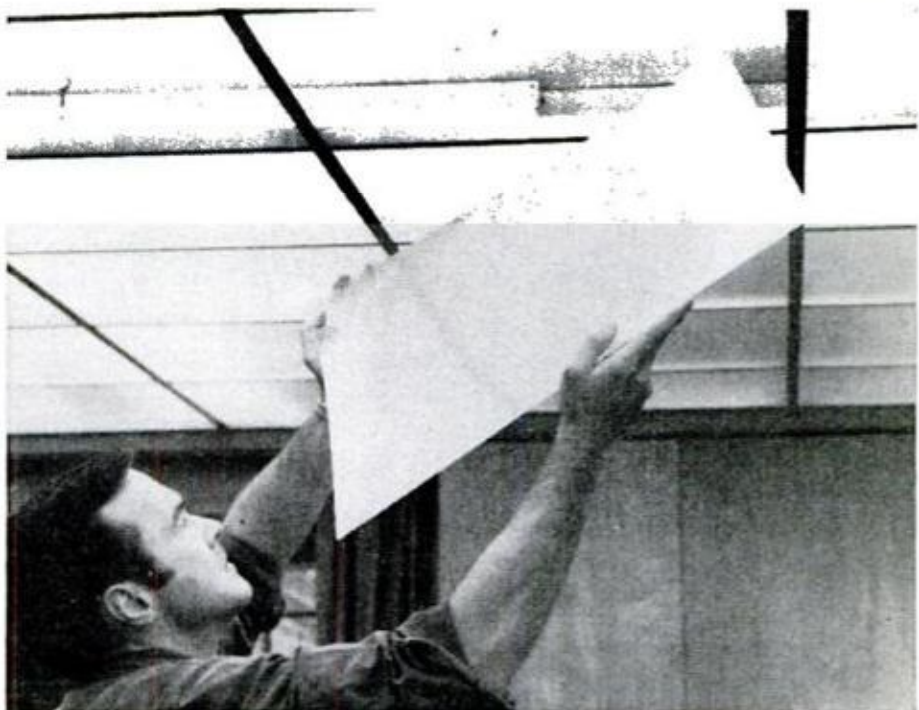
SUSPENSION WIRES (above) are cut approximately 1 in. longer than amount of drop desired and tied into tees. Hooks in the old ceiling hold other ends of the wires. Panels (below) are easily slipped into the completed gridwork
