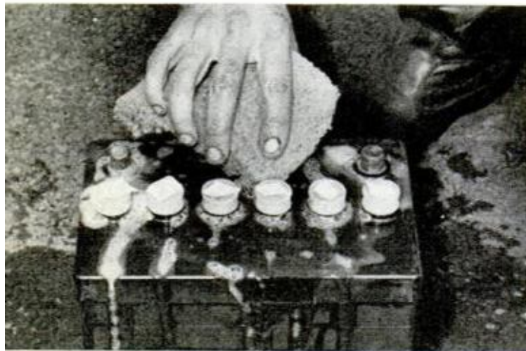
WASH ENTIRE BATTERY with baking soda solution, paying particular attention to top vents and posts
