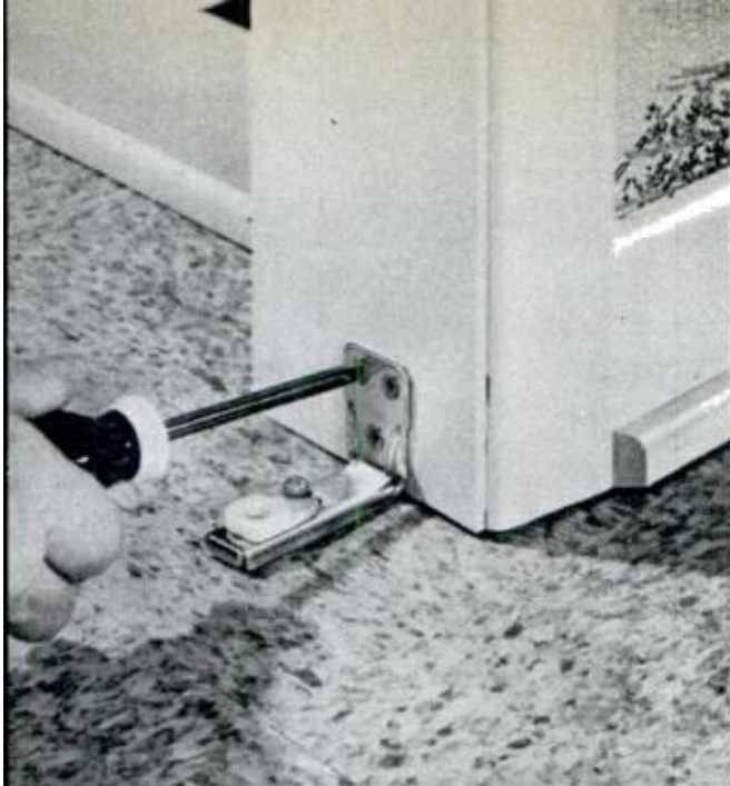
SECOND STEP: Attach the two jamb brackets at the floor and on a plumb line with the overhead track
