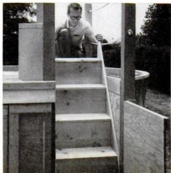
HOMEOWNER-BUILDER lowers prebuilt stairs into position. There's space at bottom for small footbath
