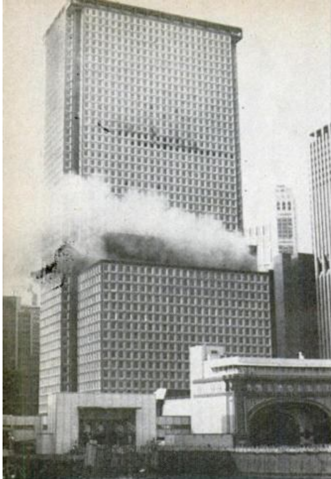
SMOKE BILLOWS around 50-story One New York Plaza as fire consumes three floors. Two died in $10-million blaze
