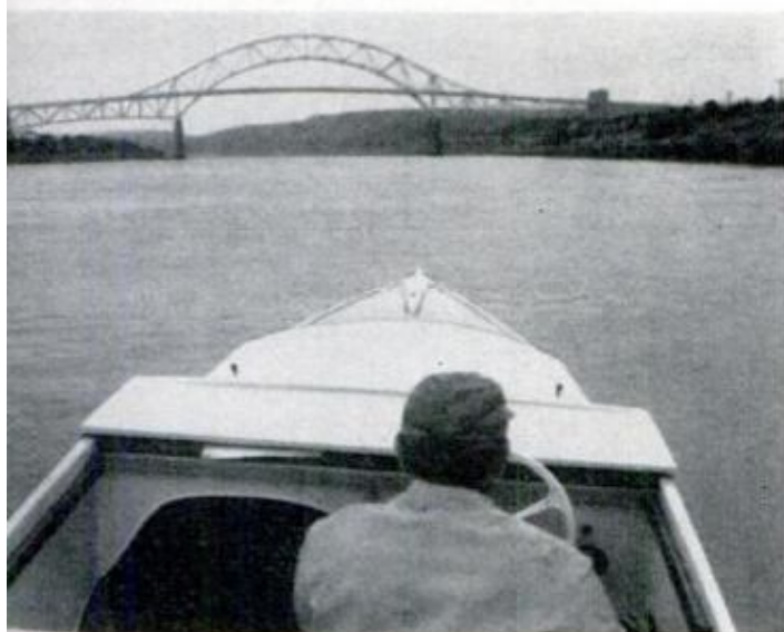
CALM OF CAPE COD CANAL , along with following tide, offered a respite from wind and storm outside
