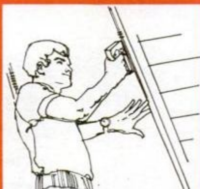
PUT UP INSULATION
