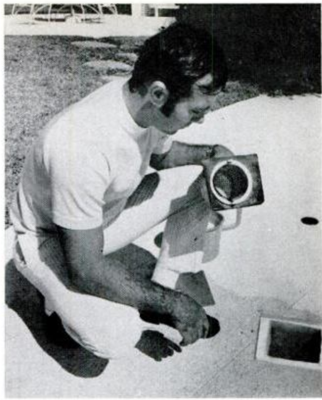
SKIMMER BASKET should be removed and cleaned. If it appears defective, replace it with a new one
