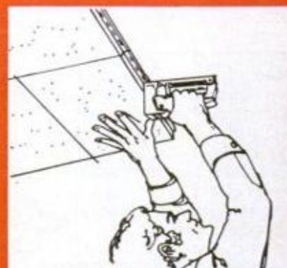
INSTALL CEILING TILE
