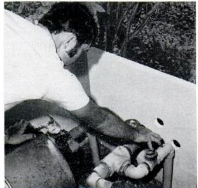
CHECK MOTOR AND ALL FITTINGS to insure that parts are leakfree; replace any defective pipe
