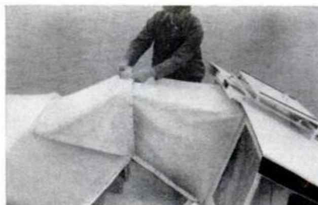
FINISHING TOUCHES are provided by the author in tying closed the little openings in mastlight seam
