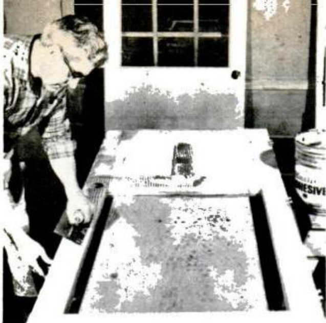
PANEL ADHESIVE simplifies facing the door interior with flush panel. Apply a thin, flat coat to door
