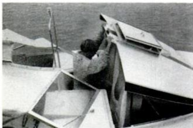
WHILE STEVE HOLDS foredeck up, Ron slides roof rods along support bars preparatory to tightening
