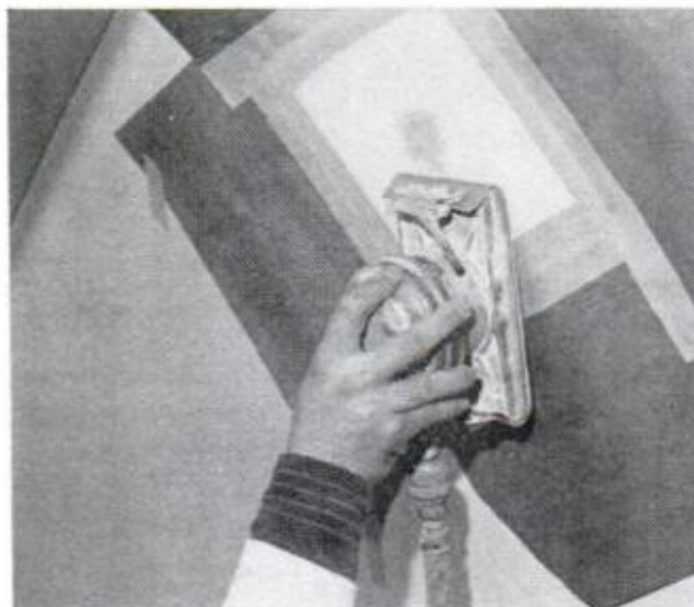
IF YOU HAVE a vibrating sander, use it. Start with 220-grit paper, wash sanded area frequently with water as you work to keep repair zone free of dust
