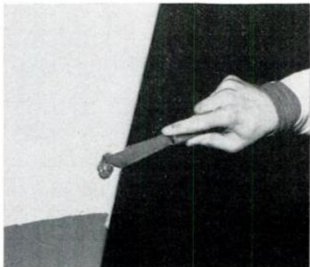
REPAIR PUTTY must have a firm seat on which to hold, so scrape away all loose distressed material
