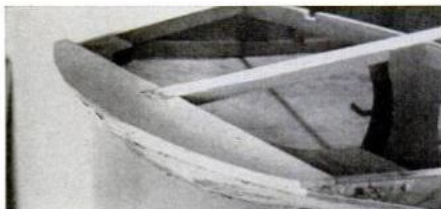
PINE BLOCKING needed on bow extends from sheer to sheer, must be faired to form crown of decking
