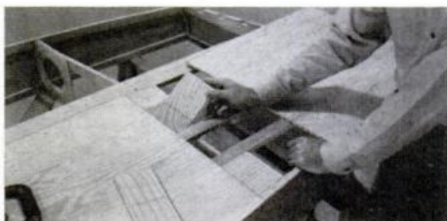
BUTT-BLOCKS are fitted between the battens before the planking is permanently fastened to hull
