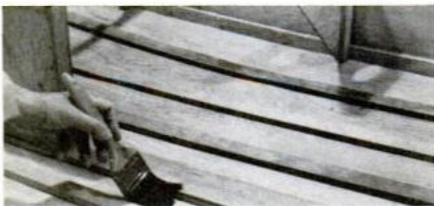
INTERIOR of the boat should be painted prior to applying the decking. Use a quality marine paint
