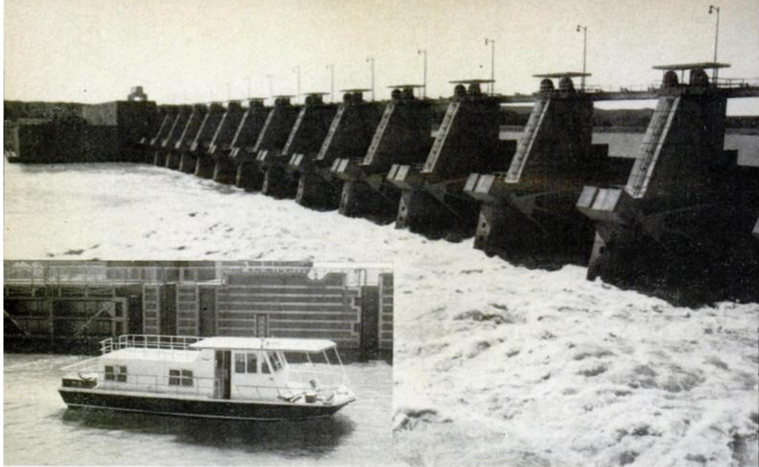
TUMBLING TORRENTS below dams are in striking contrast to the quiet rise of water in the locks
