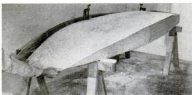
BATTENS ARE NOTCHED into transom and rest on the frame. Next, bottom panel is trimmed in place
