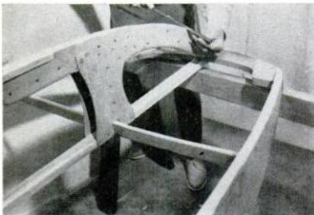
FAIRING is started by filing a series of equally spaced grooves all along the stem, keel and chine
