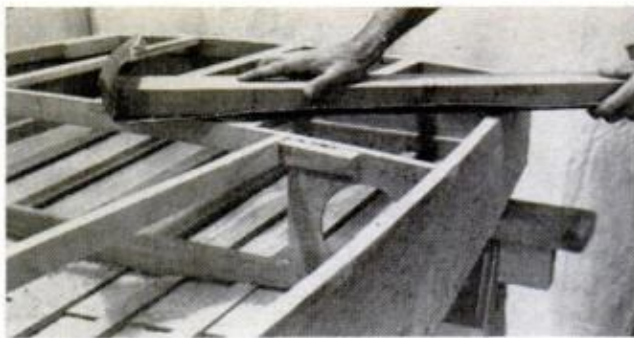
GOOD METHOD of insuring a smooth fairing job on aft section is sandpaper glued to a length of 2x4
