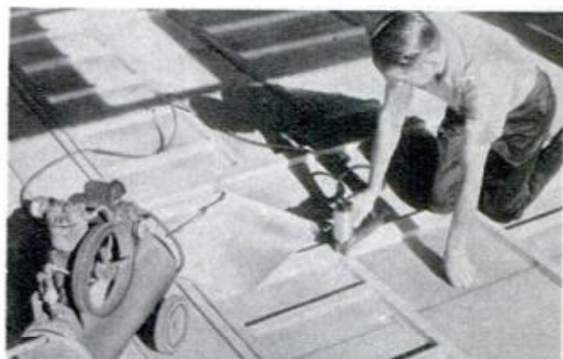
SIDEWALLS ARE FRAMED on shop floor. Jig for framing is made on 1/2-in. plywood later used for floor
