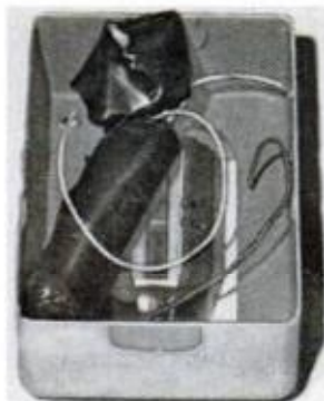
ELECTRICAL OUTLET in office of Wall Street firm contained a "bug" (right) hooked to tape recorder
