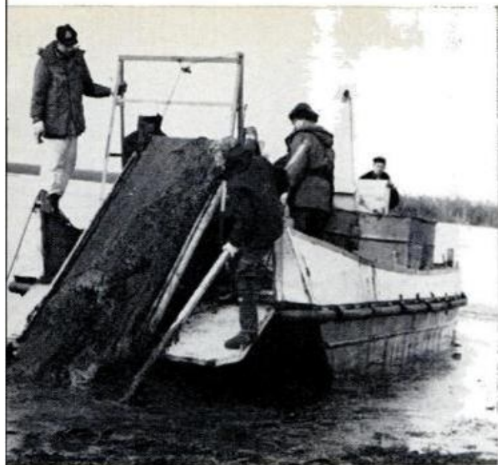
OILEVATORS WERE USED to sop up oil off Nova Scotia after tanker Arrow ran aground and broke up
