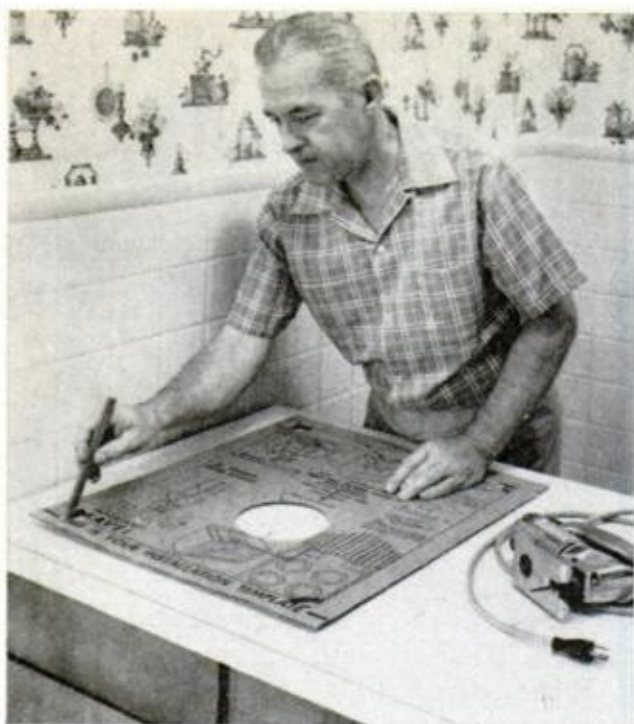
1. USING TEMPLATE that comes with grill, place it in position on counter and pencil-mark four corners
