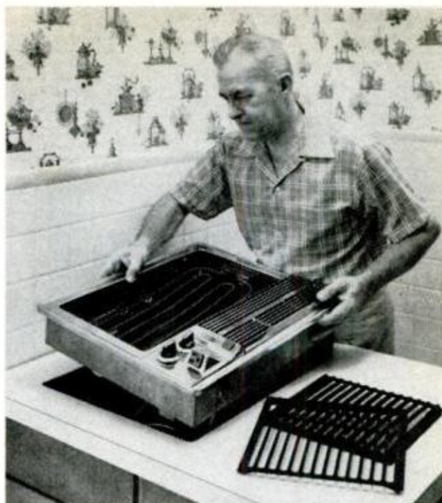
4. WITH DUCTWORK IN PLACE , lower grill in cutout and connect to pipe. Then screw in glass grease jar
