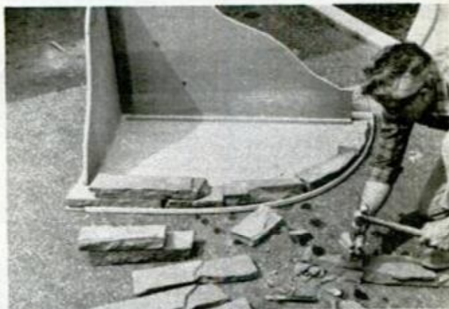
BLUESTONE can be cut with chisel, but buy a few extra pieces. Chalk-number pieces as they are fitted
