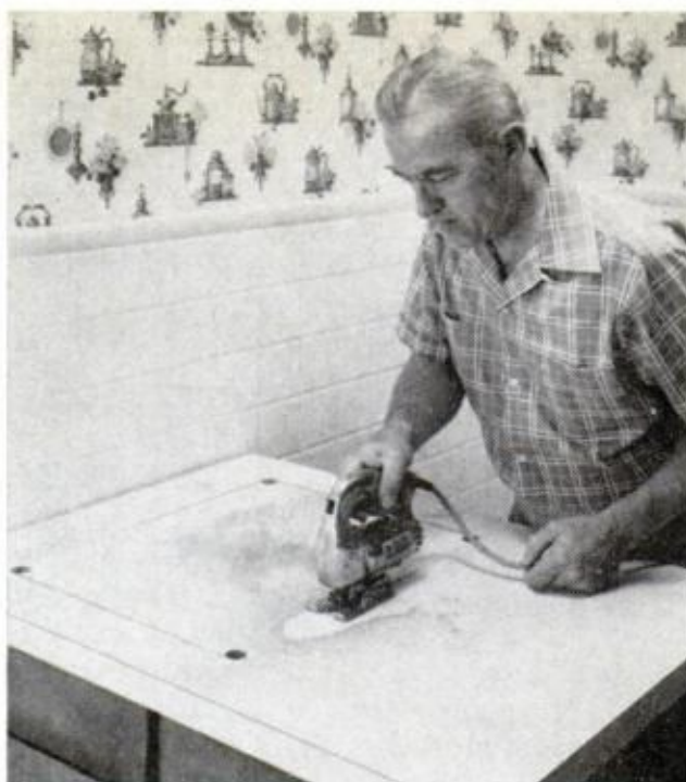
2. AFTER DRAWING LINES from corner marks, bore holes and carefully saw along lines with a sabre saw
