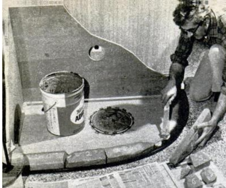
PANEL ADHESIVE holds first course of stone to the wood. For convenience, prepaint base edge first
