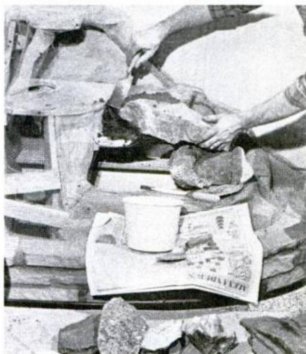
USE STIFF MIX but dampen rocks to insure a good bond. Compact the mortar so it will be watertight
