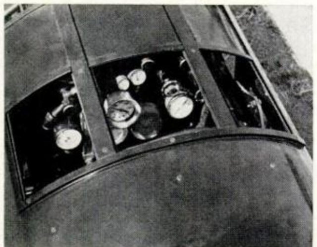
FROM ENGINEER'S SEAT aboard tender, Mann can see this array of tiny pressure and steam gauges
