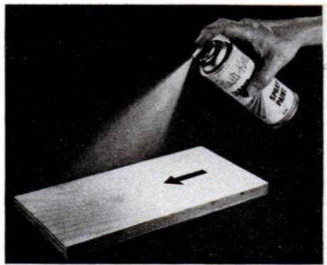
WORK AWAY when spraying flat surface so over-spray (mist) settles ahead of full wet coat following
