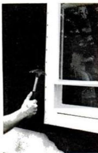
WINDOW INSTALLATION is simple; plastic "fins" that you insert into the side jambs are provided with holes for use in nailing to sheathing. To prevent leaks, felt is stapled over the fins. Clapboard, which follows, finishes exterior
