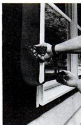
WINDOW INSTALLATION is simple; plastic "fins" that you insert into the side jambs are provided with holes for use in nailing to sheathing. To prevent leaks, felt is stapled over the fins. Clapboard, which follows, finishes exterior
