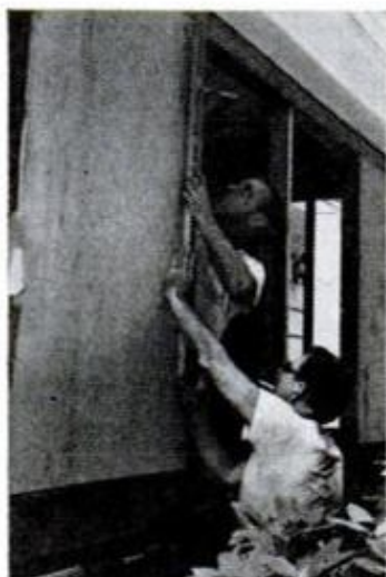
ROUGH OPENING is measured for new framing (left); exterior sheathing is applied next. Small opening in background (right) is framed for windows, which go in next. Windows here were installed with one stud between them
