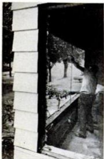
ROUGH OPENING is measured for new framing (left); exterior sheathing is applied next. Small opening in background (right) is framed for windows, which go in next. Windows here were installed with one stud between them
