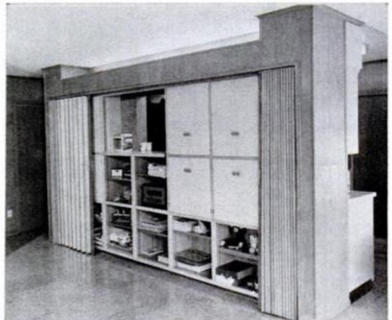
FULL-DEPTH WALL gives that ample storage so much appreciated by a large family. Accordion doors hide it all when desired
