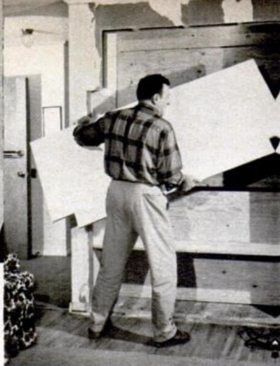
BACK OF CLOSET is ripped out and \frac{3}{4} -in. plywood is nailed to back edge of the doorjamb. The cabinet (above) is framed and Formica countertop installed, using screws and corner braces
