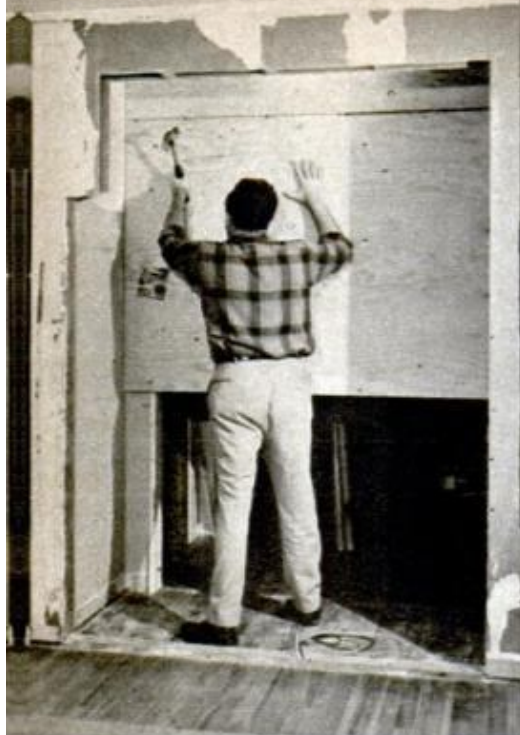
BACK OF CLOSET is ripped out and \frac{3}{4} -in. plywood is nailed to back edge of the doorjamb. The cabinet (above) is framed and Formica countertop installed, using screws and corner braces
