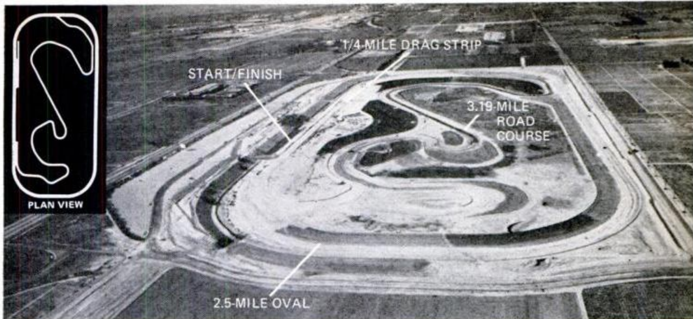
THREE-IN-ONE FACILITY includes drag strip and road circuits as part of the oval. Back straight is 30 feet higher than front straight; first row of stands is 30 feet above track for 100-percent viewing of the oval
