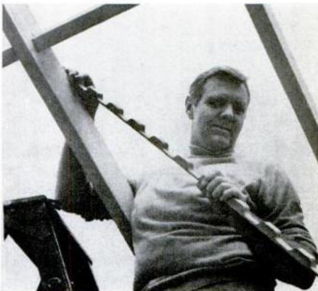
CONFIGURED FILLER STRIPS are nailed atop cross braces, provide solid nailing (below) for panels
