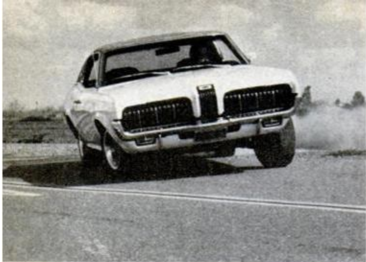
COMPETITION HANDLING PACKAGE costs $31, adds to cornering power but makes soft ride a bit harsh
