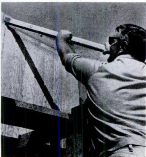
CROSS BRACE is installed flush with top of rafter. Diagonal brace (below) keeps the structure square
