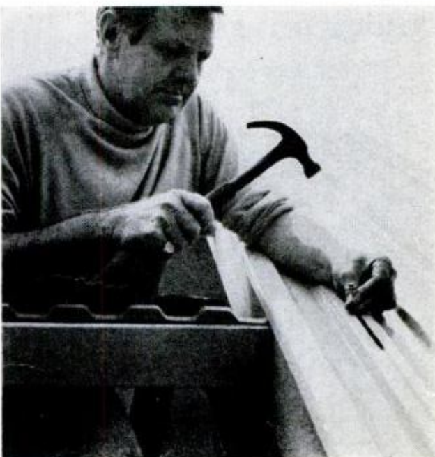
CONFIGURED FILLER STRIPS are nailed atop cross braces, provide solid nailing (below) for panels
