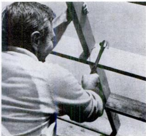
CROSS BRACE is installed flush with top of rafter. Diagonal brace (below) keeps the structure square
