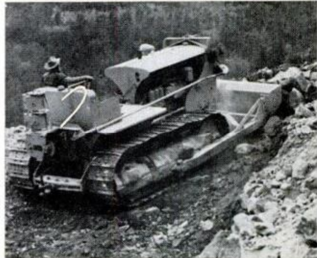
PROGRESS is "mucking" blasted rock off the mountain with a big "cat" after years of doing it by hand
