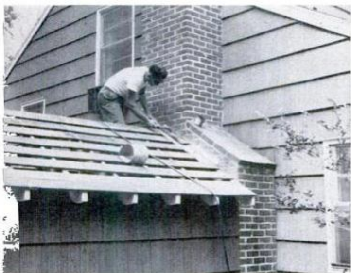
TO INSURE DRY FIREWOOD , roof was carefully flashed where it meets chimney and 15-lb. felt was stapled over upper 10 in. of each course of shingles JUNE 1970
