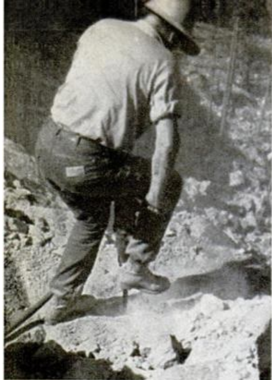
DRILLING PROGRESS: In the early '50s, Ziolkowski and a hired man were "leaning" on 115-p.s.i. jackhammers (left) to average 40 feet a day. Twelve years later, he hauled a wagon drill up the mountain and boosted rate to 200 feet a day. Sculptor's sons now operate self-propelled Air-Trac rig (right) at rate of a foot a minute
