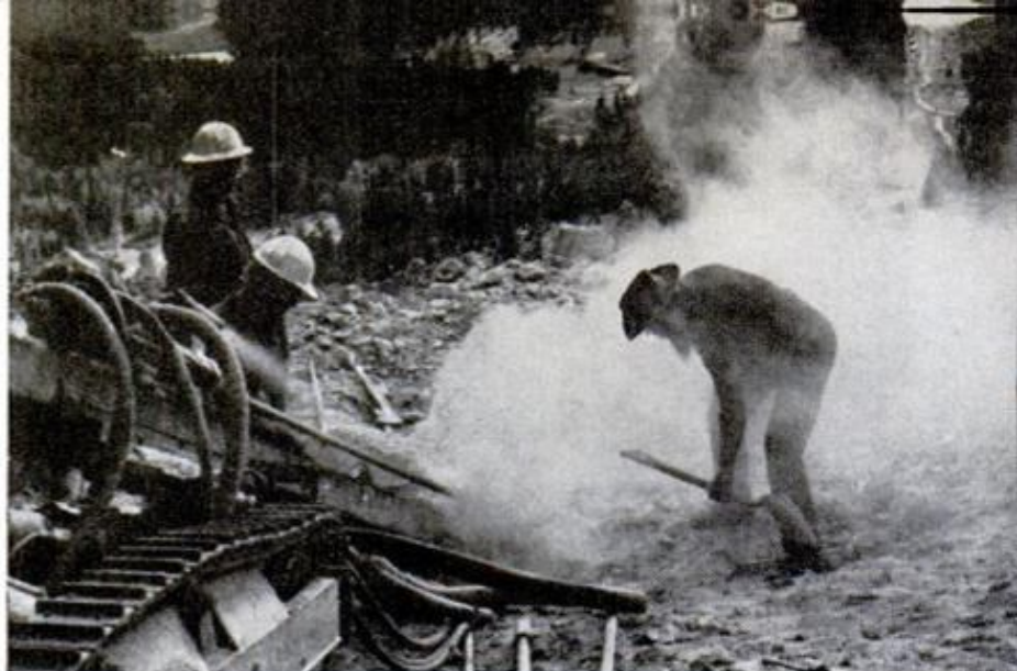
DRILLING PROGRESS: In the early '50s, Ziolkowski and a hired man were "leaning" on 115-p.s.i. jackhammers (left) to average 40 feet a day. Twelve years later, he hauled a wagon drill up the mountain and boosted rate to 200 feet a day. Sculptor's sons now operate self-propelled Air-Trac rig (right) at rate of a foot a minute
