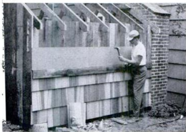
FIBER BACKER-BOARD is placed as an overlap above each course of shakes. It produces offset and architectural shadowlines at butt edge of the shingles
