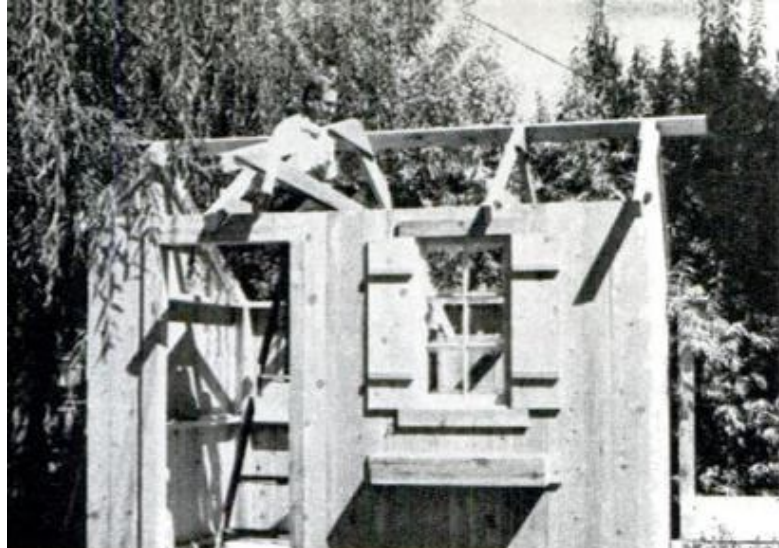
PREASSEMBLED ROOF FRAMING is hoisted into place and fastened to 1x6 ridge board installed at the peak
