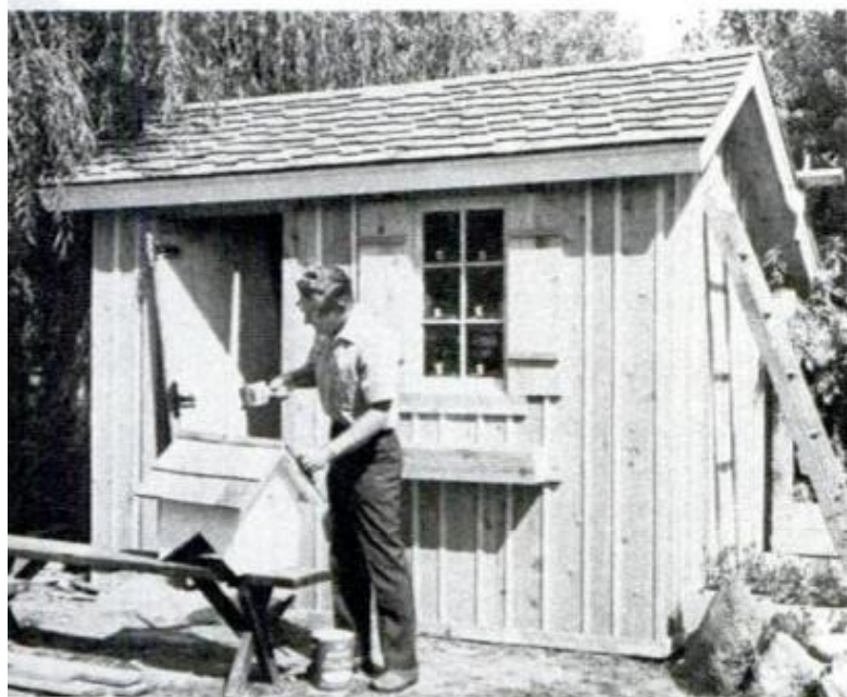
ROOF SHINGLES are laid 5 in. exposed to weather; 3/4-in. exterior-plywood door is hung with T-hinges
