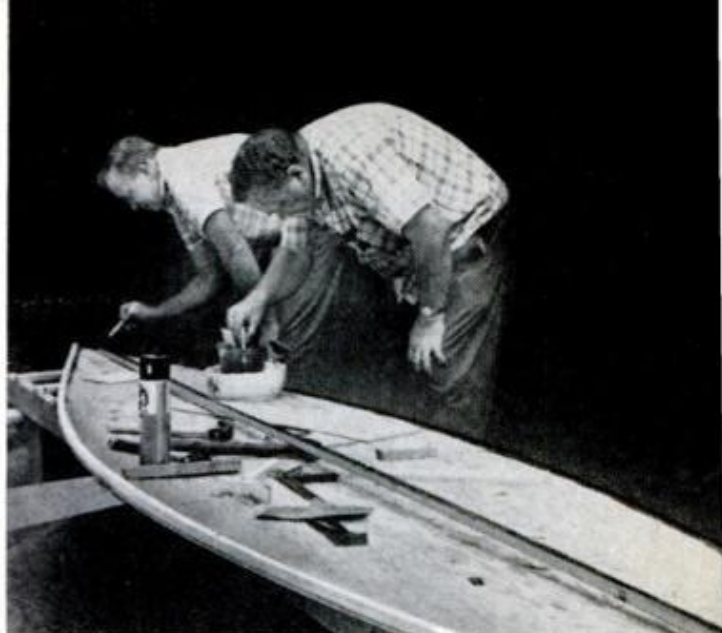
REST BOTTOM PANELS (still joined) on raised surface; glue and nail chines in place along edges
