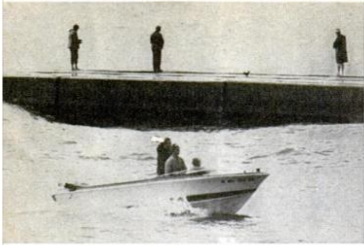
A BREAKWATER that opens directly onto ocean or a big lake may be troubled by surges and heavy swells
