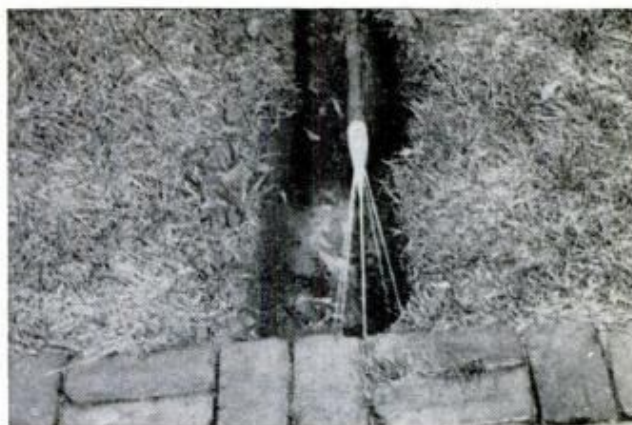
PLACED IN TRENCH, pipe (left), is forced through soil under walk using water pressure (above). Placement is completed (below) and nozzle is removed
