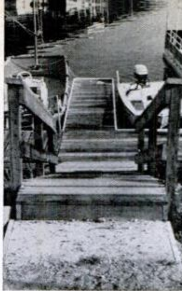
GOOD MARINAS provide protective handrails for their stairs, adequate maneuvering room near slips and strong, yet neat, fendering along the docks
