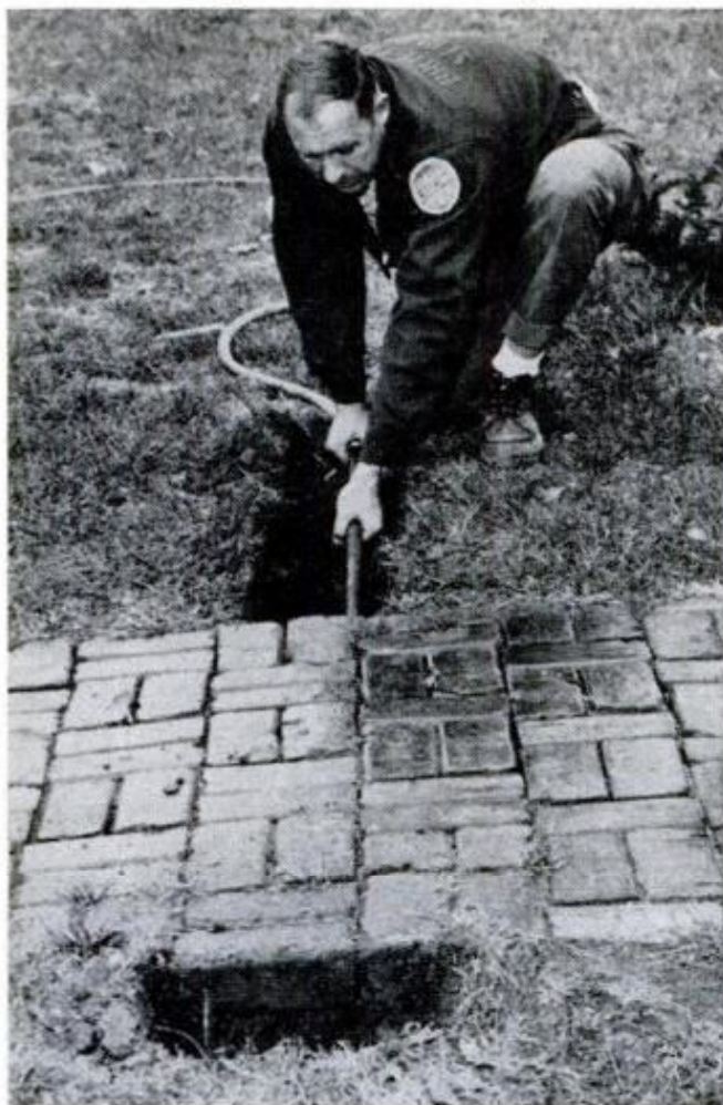
PLACED IN TRENCH, pipe (left), is forced through soil under walk using water pressure (above). Placement is completed (below) and nozzle is removed
