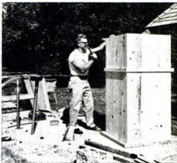
BOX-LIKE FLUE is made with 1x6 V-groove boards, shoved up through roof collar, nailed
