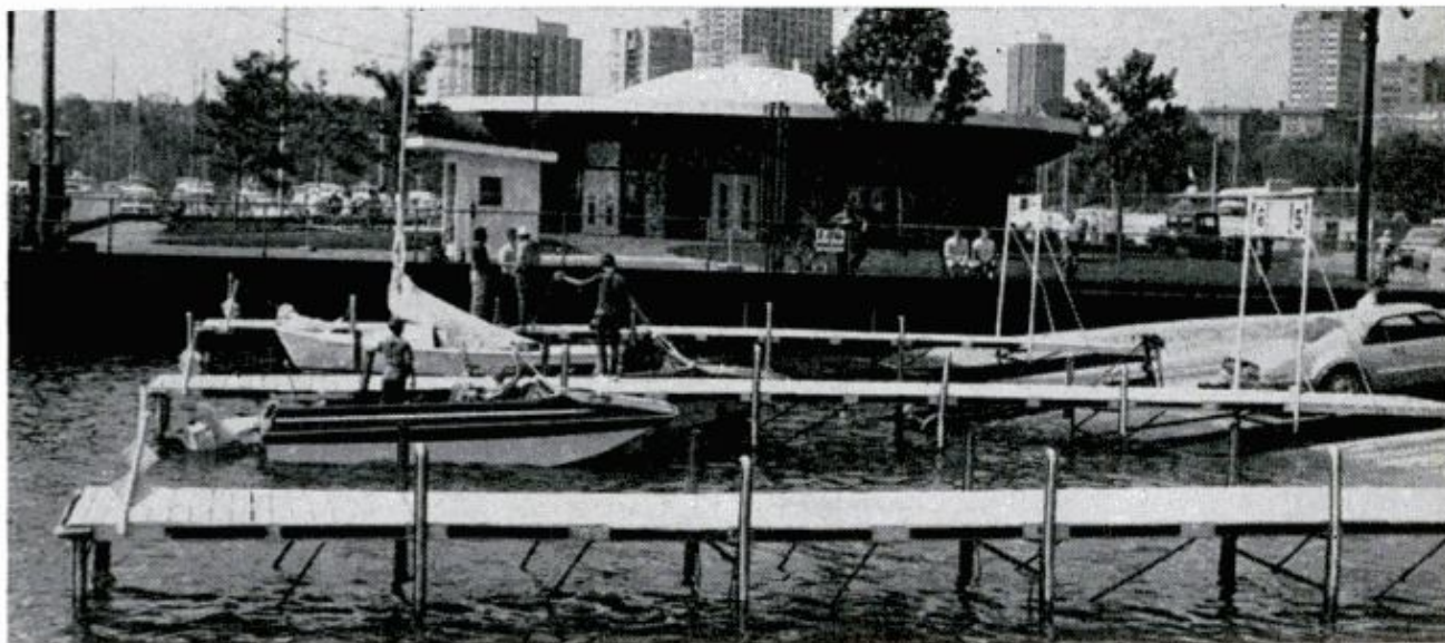
LONG DOCKS in launching zone allow one boat to continue outfitting while another is launched in front of it
