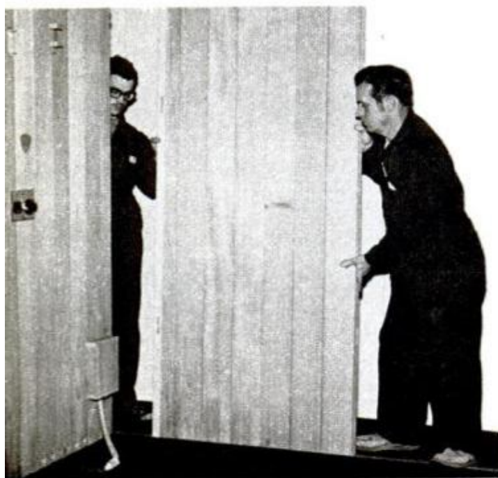
WALL SECTIONS , redwood on inside, mahogany outside, come insulated and designed to hook together
