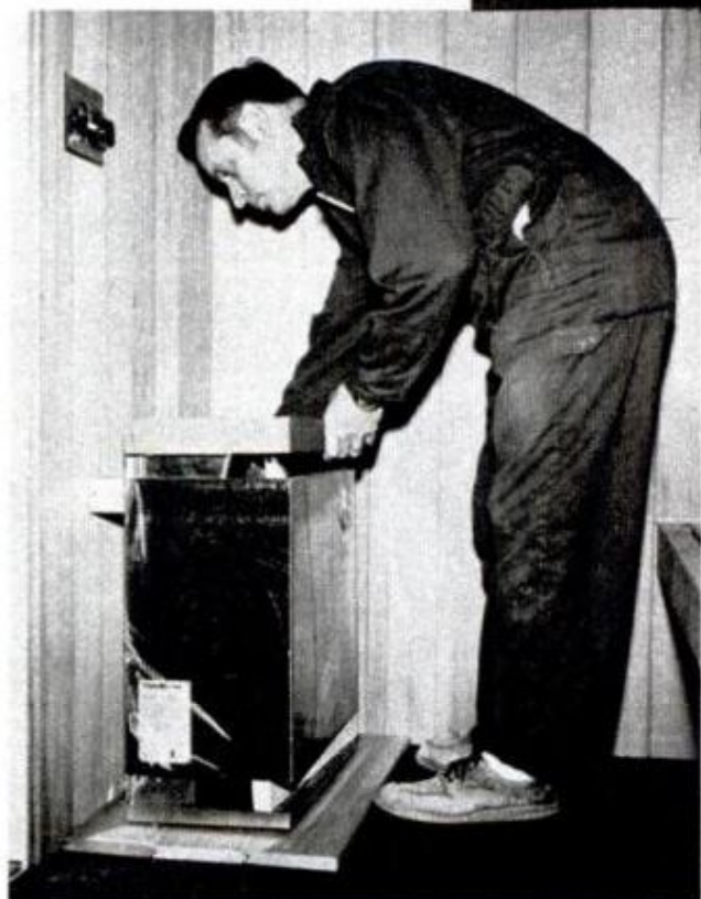
FINALLY, ELECTRIC HEATER is placed in corner and fenced-in by picket enclosure. Heater runs noiselessly
