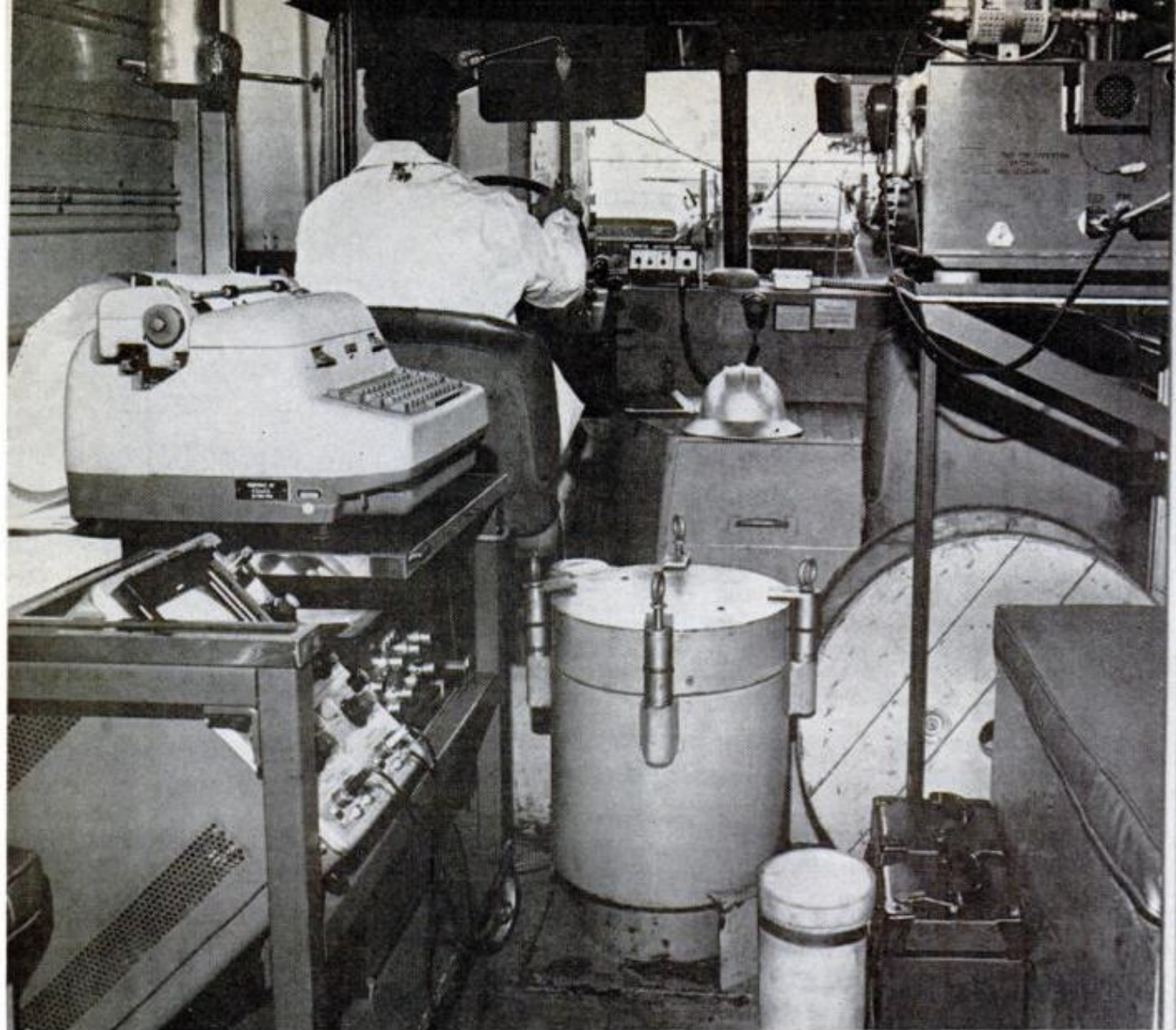
INSIDE EMERGENCY VAN is lead-shielded gamma "well" (large cylinder) into which samples are placed for analysis. Multichannel analyzer (left) gives a printout of analysis. Oscilloscope (resembling TV screen) shows spectrum, helps identify radio nuclei. Electronic gear (right) is radio communications equipment
