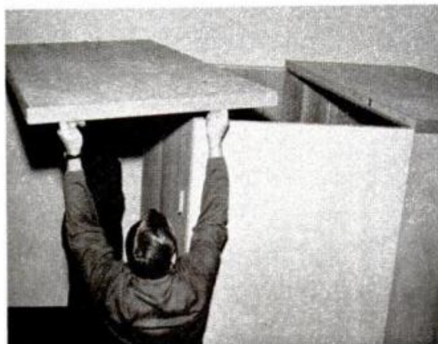
SAME LOCKING METHOD is used to clamp ceiling panels in place. Panels are treated against warping
