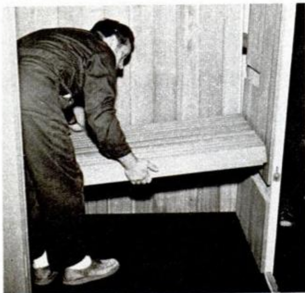
OPEN-SLAT BENCHES of kiln-dried redwood come ready-built, never become uncomfortably hot to touch
