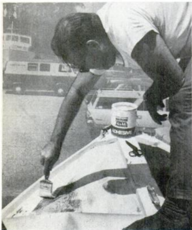
ADHESIVE RESEMBLES WHITE GLUE. Two coats are applied with a brush to insure a thick covering. Work small sections at a time, starting at the center
