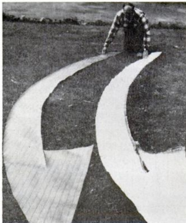
RESULTING ONE-PIECE HALF-DECKING is duplicate of the worn-out surface it replaces at right. Fit is exact; material closely simulates the planking
