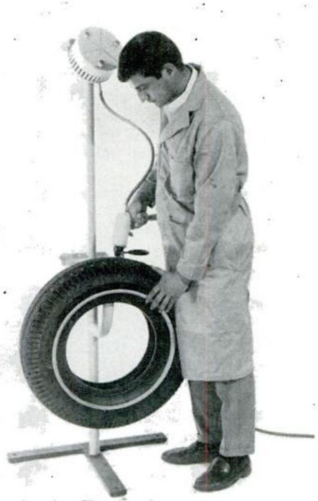
STUDS ARE INSERTED with compressed air gun. Stud gun fingers spread pinhole (top). When trigger is squeezed, a piston advances, driving stud into hole. Professional studding equipment (right) is needed
