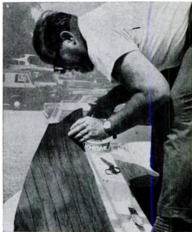
COTTON-FABRIC-BACKED DECKING has good body and handles easily without stretching. Glue used dries transparent and leaves no ugly splashes or spots
