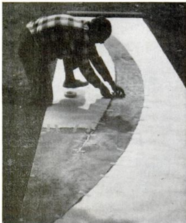
FIRST STEP is to remove old canvas decking carefully. Next, it is taped face down on the back of the new vinyl to serve as an exact cutting pattern
