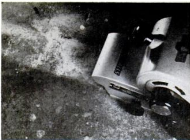
CONCRETE FLOOR STAINS can be cleaned with a belt sander. Tool's not limited to wood and metal chores
