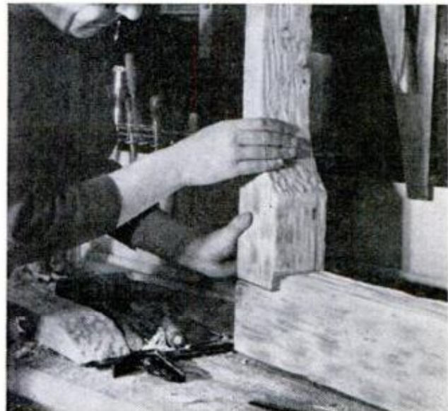
KNEE IS PERMANENTLY ATTACHED to main beam with glue and dowels before the beam is installed
