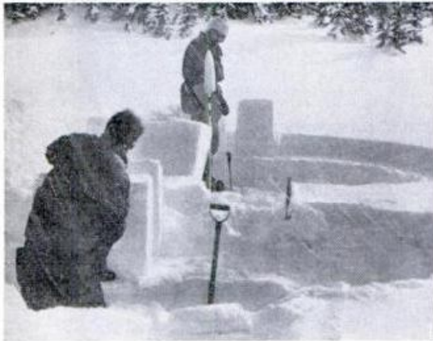
OUTSIDE IGLOO'S PERIMETER , snow blocks are taken from a "quarry" which will later become entrance
