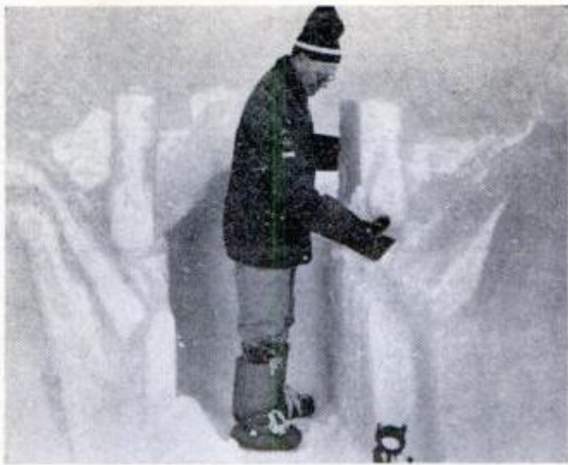
SNOW CAVE 8 to 10 feet deep built with 36-inch-long blocks is the simplest survival shelter to make
