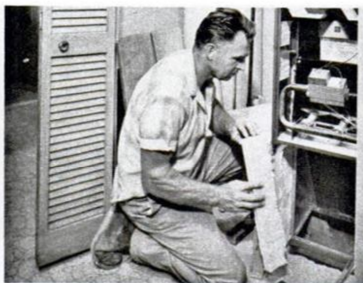
UTILITY ROOM DOORS open full width of wall for easy access when servicing furnace and water heater
