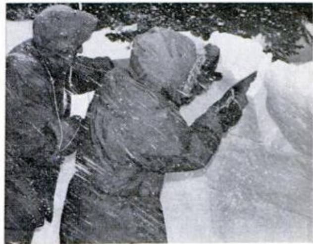
EACH LAYER OF BLOCKS leans increasingly inward. Saw is used to shape and fit blocks together
