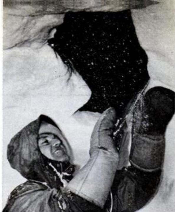
AUTHOR ENTERS IGLOO through passage 6 feet below floor level. This corridor keeps wind out; warmth in
