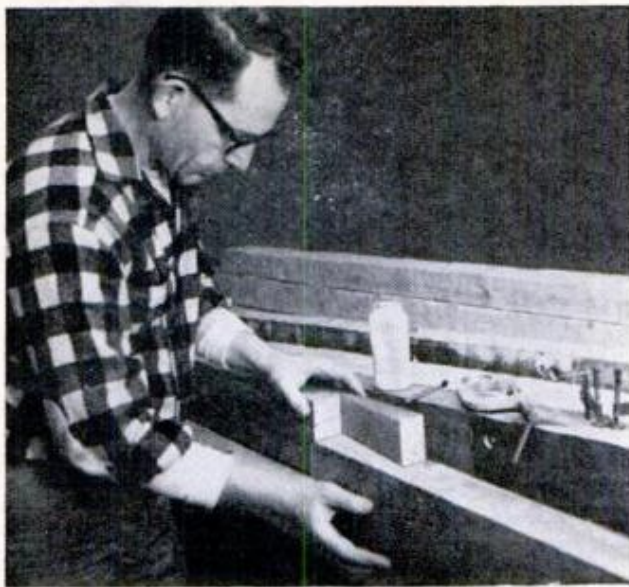
BEVELED SPLICES ARE CHECKED to insure fit, then assembled, using glue, lagscrews and dowel-plugs
