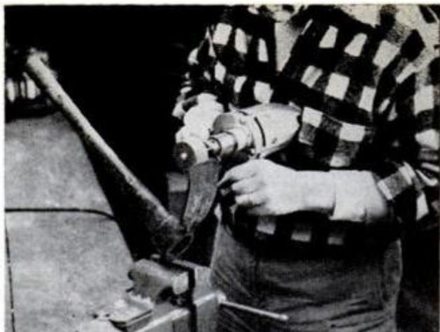
SURPLUS PICK-MATTOCK is rough-ground into an adz, using portable grinder. Bevel is on the inside
