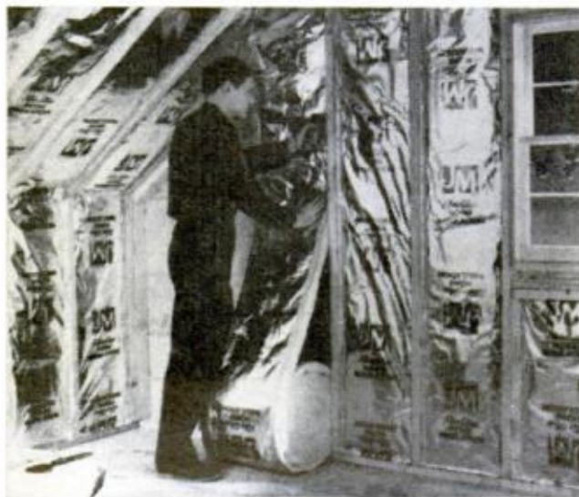
FOIL-FACED insulations are stapled to stud sides to provide air space between foil and back of wall
