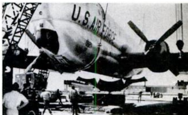
SUPPORTED BY FIVE CRANES , KC-97 dangles as transporter (with nose yoke open) is slid under plane
