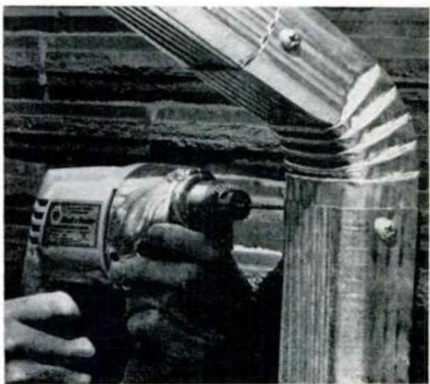
ELBOWS are used to bring the leader back from the roof overhang to a downspout on the house wall. After positioning, holes are drilled for the rivets
