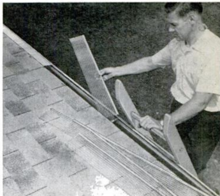
LEAF GUARDS in strip form fit between shingles and gutter bead, keep gutter free of debris accumulation
