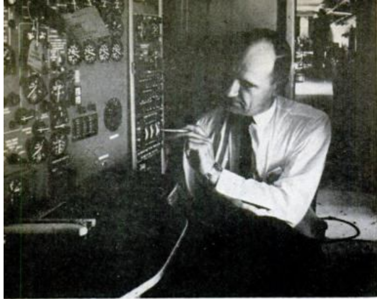
CAT INDICATOR IS INSTALLED on engineer's panel of Pan Am 707. When indicator shows a sudden temperature change, crew knows CAT may be ahead
