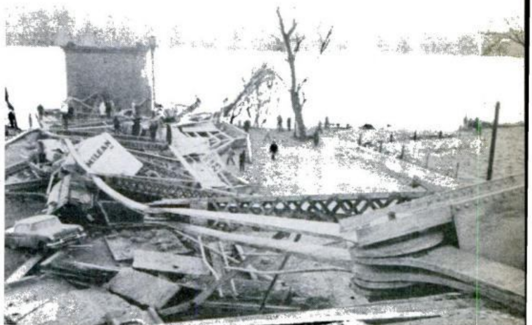
SMASHED CARS AND TRUCKS lie in the twisted wreckage of the Silver Bridge, which collapsed shortly before Christmas in 1967, killing 46. Spanning the Ohio River near Point Pleasant, W. Va., the structure is believed to have failed because a connecting pin gave way. One of these pins, joining several bridge links, can be seen in the foreground at right. Modern testing methods using NDT principles make a repetition of such a disaster unlikely
