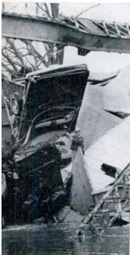
SMASHED CARS AND TRUCKS lie in the twisted wreckage of the Silver Bridge, which collapsed shortly before Christmas in 1967, killing 46. Spanning the Ohio River near Point Pleasant, W. Va., the structure is believed to have failed because a connecting pin gave way. One of these pins, joining several bridge links, can be seen in the foreground at right. Modern testing methods using NDT principles make a repetition of such a disaster unlikely
