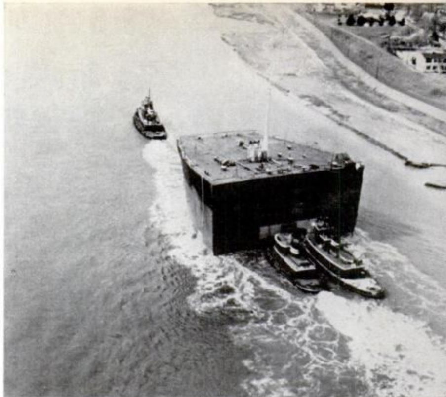
BIG HUNK OF SHIP —the Manhattan's forward section—leaves for Newport News, Va., yard. New ice-breaking bow (see drawing) was built in two parts
