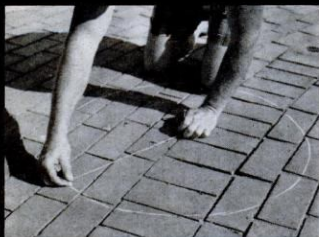
FIRST DRIVE NAIL and swing 30-inch circle with chalk and string. Bricks are placed around the circle
