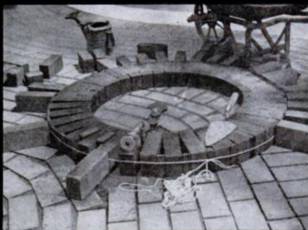
BRICKS ARE SPACED at outer edge by inserting wood spacers, then tying the circle of bricks with cord
