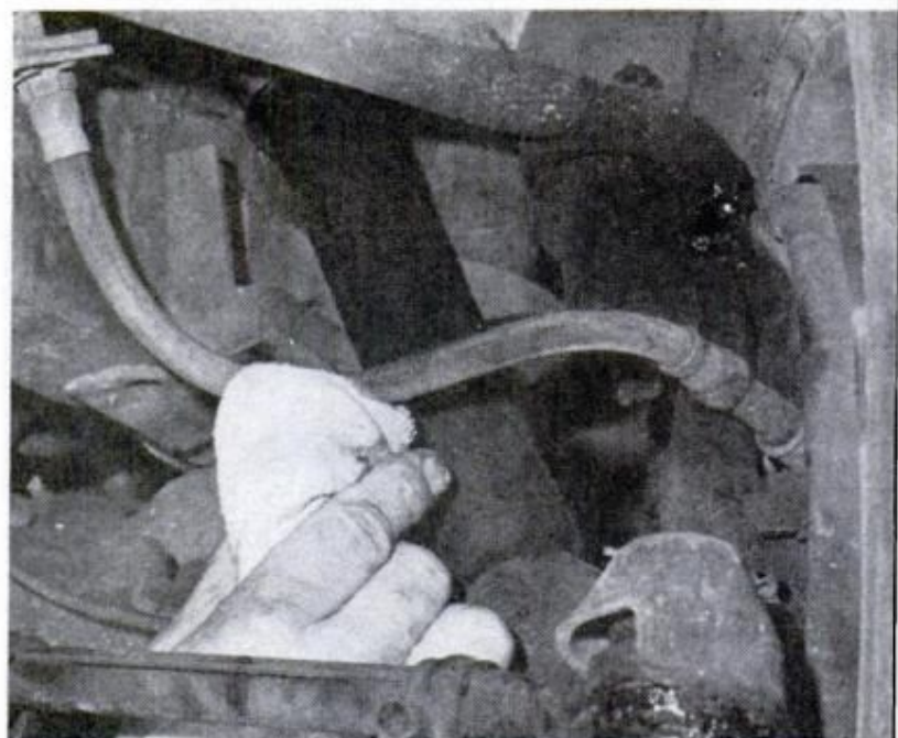
BRAKE HOSES are exposed to hazards of the road and should be wiped down and checked periodically. This examination should be considered a supplement to a good habit of looking over garage floor for possible leaks of fluid (which also has a distinctive and easily detectable smell)
