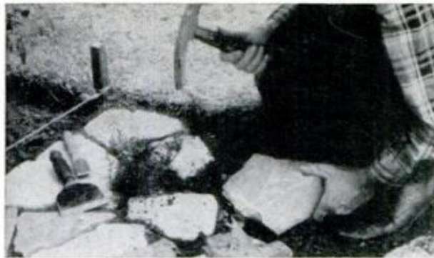
IF NECESSARY , you can chip stone to fit awkward-shaped areas, but always wear safety goggles
