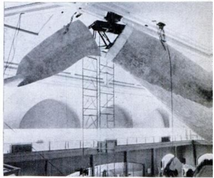
6 LOCKING DEVICE is used to bring together 28-foot tail and 66-foot body. Mechanism connects to steel pipe anchored in reinforced ceiling
