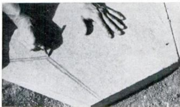
WHERE A BLOCK MUST BE CUT , make a pair of guide lines, each about \frac{1}{4} -in. off desired cutline
