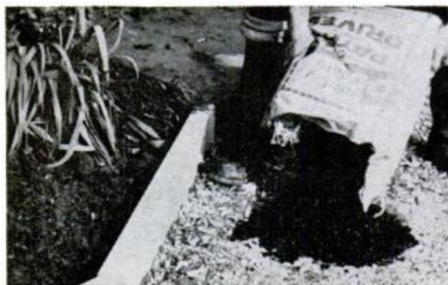
BREAK OPEN the bags of asphalt and pour this on top of gravel bed. Asphalt comes in several colors
