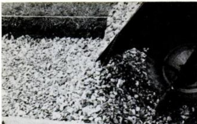
POUR A GENEROUS AMOUNT of gravel on top of a firm foundation and rake it until it's spread evenly
