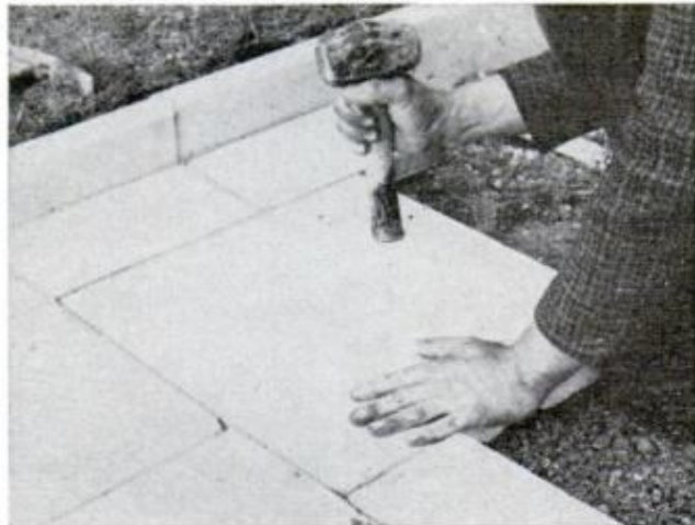
TAMP THE SLAB firmly into place by using the handle of a hammer—never pound it with hammer's head
