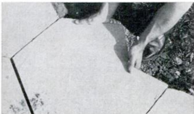
LOWER THE CUT BLOCK gingerly into place on the bed, making sure that the smooth bed isn't disturbed
