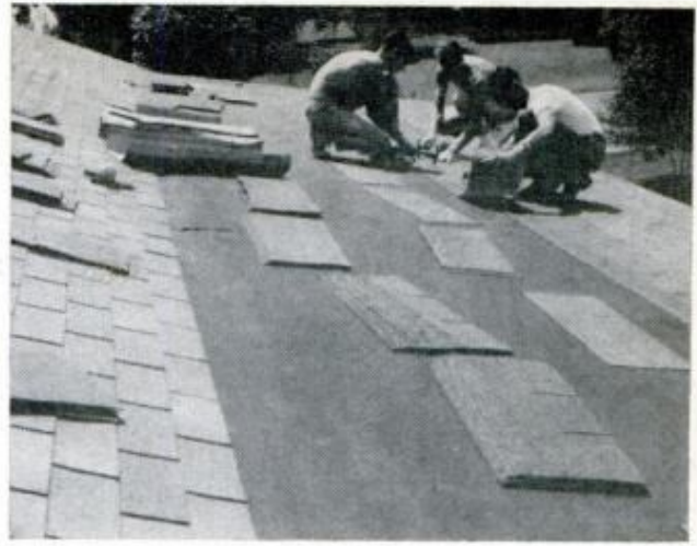
AFTER ADDING FLASHING , roof sheathing is covered with building felt and matching shingles are applied
