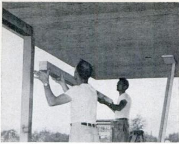
PERMANENT 4x4 POSTS are anchored to slab with angle brackets, then a 4x4 lintel is placed on top
