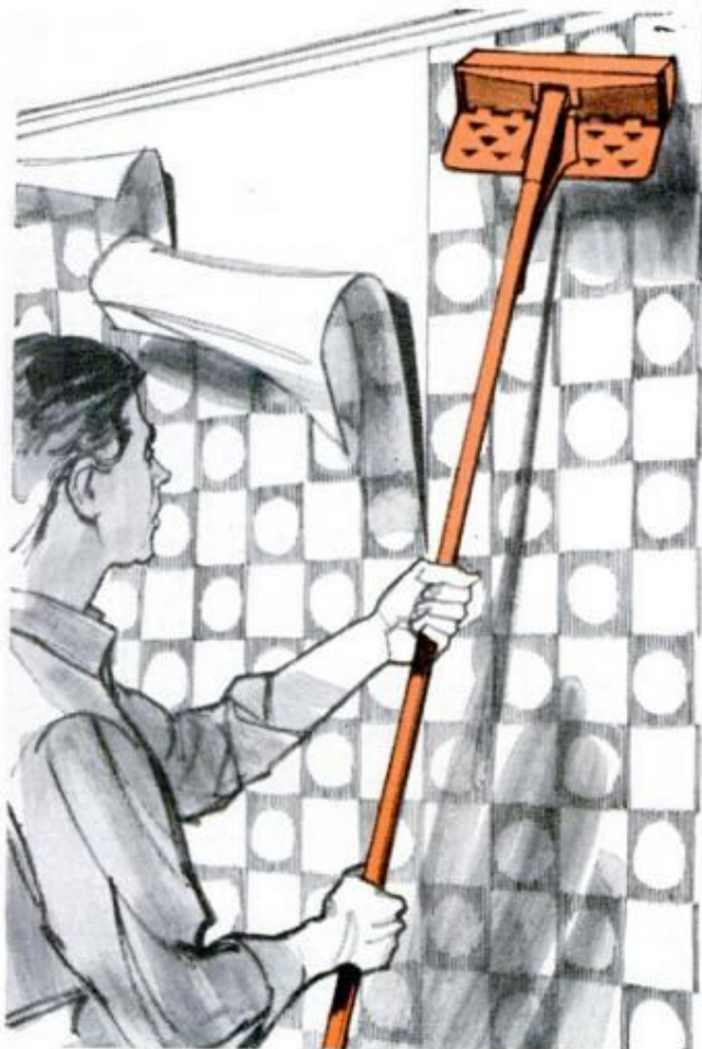
SPONGE-TYPE FLOOR MOP can help make quick work of removing wallpaper, since you can use hotter water than you would by hand. Ladder isn't needed
