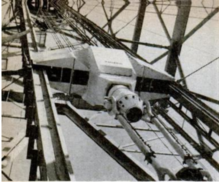
DRILL RIG towers above deck. Crown block rides between two guide beams and supports drill string
