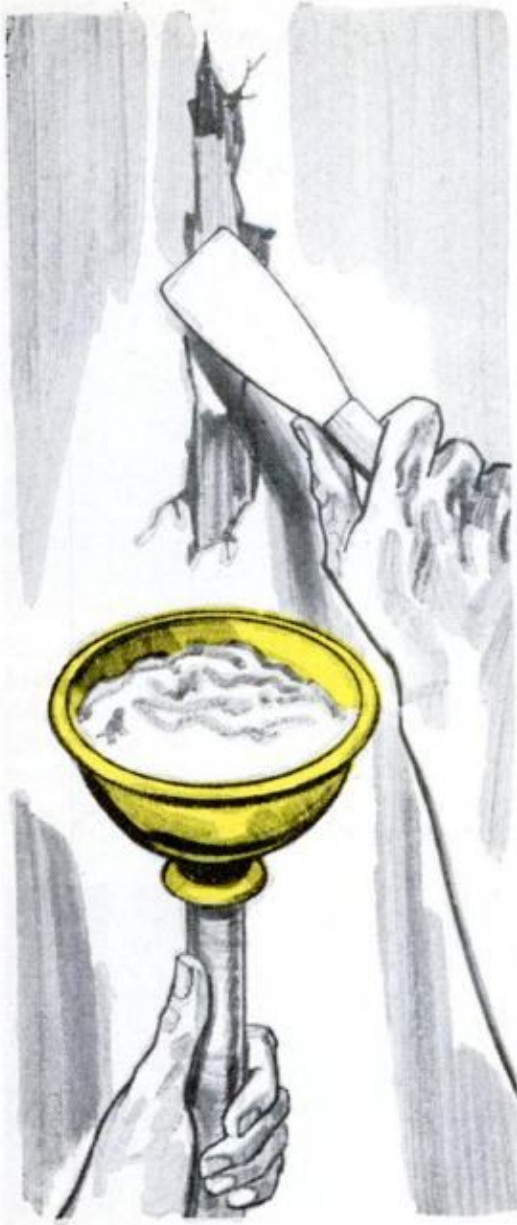
PLUMBER'S FRIEND makes a good mixing container for small batches of spackling compound. It's handy to hold, and the flexible cup is easy to clean, even if some of the plaster should become hard
