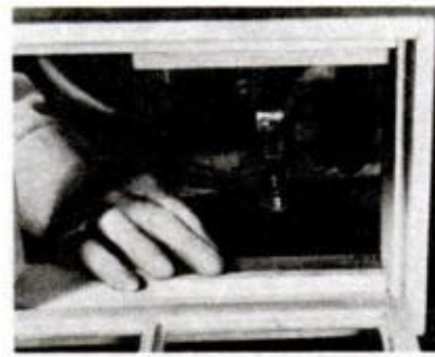
MAGNETIC CATCH , stripped of its frame, is fastened to case with screw through center hole
