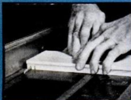
SECOND CUT more than halfway to end is then made and area between cuts is cleaned with saw.
