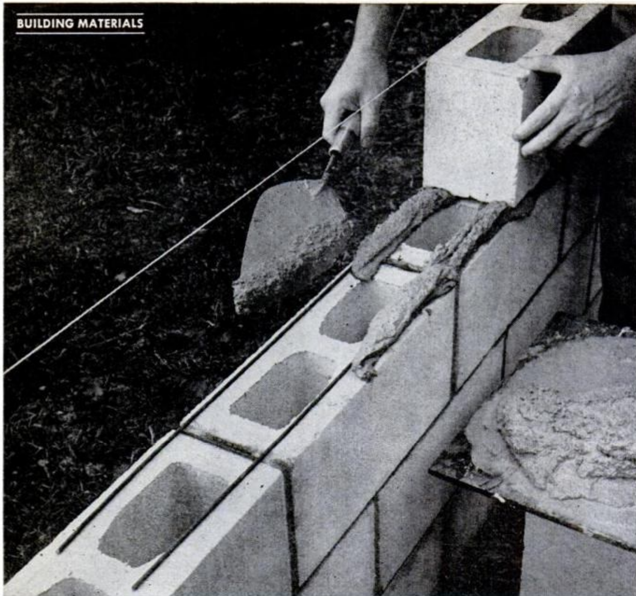
EASIEST REINFORCEMENT to install is steel block mesh set in mortar. Ends of mesh strips are overlapped
