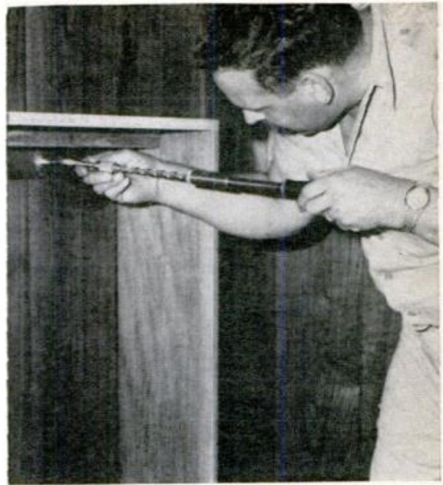
BED CABINET PROPER is anchored to wall and studs first by driving screws through top and bottom cleats
