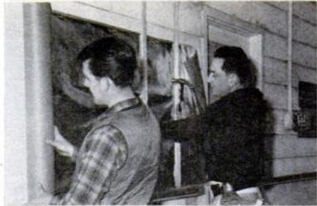
LAYER OF FOIL under the siding protects against condensation. Vertical laths bridge old lapped siding
