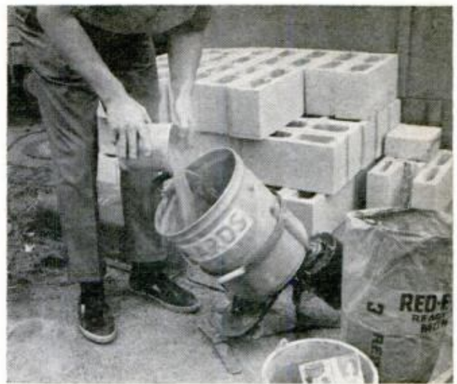
SMALL CONCRETE MIXER makes it possible to mix fresh batch of mortar while you are using up first
