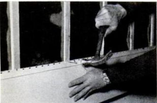
SIDING IS NAILED to the lath. It's important that you leave 1/32-in. gap between nailhead and crown
