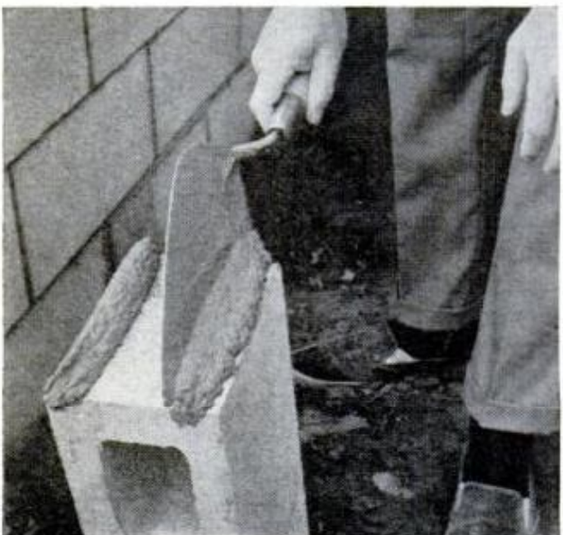
RIBBONS OF MORTAR on ends of each intermediate block fill vertical joints. For best bond, slap them on
