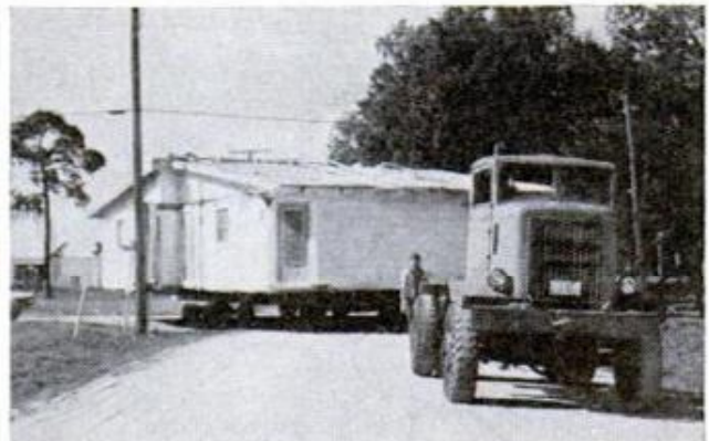
inched gradually around by winches. Wheels on inside of turn are blocked stationary so that load pivots on them, swinging around on the outer wheels
