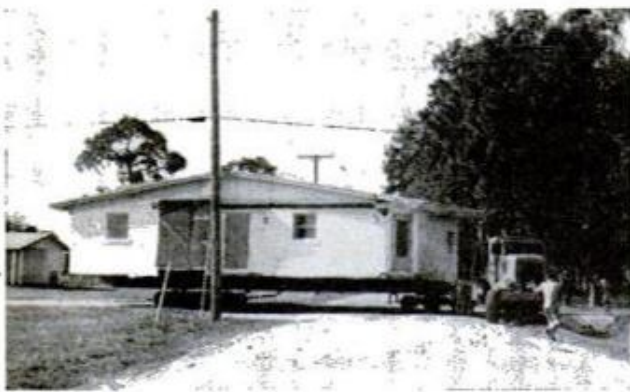
WILL IT MAKE IT? Negotiating a seemingly impossible turn calls for tricky maneuvering. Tractor must be unhitched, as shown at right, and the house
