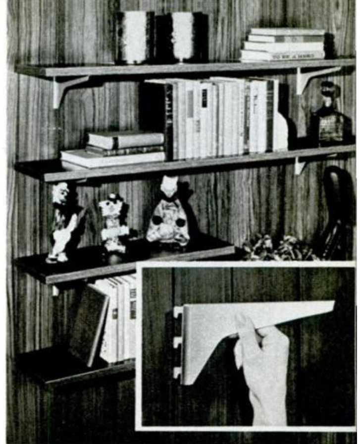
SLOTS IN THE GROOVES of special paneling take place of standards to support brackets and shelves
