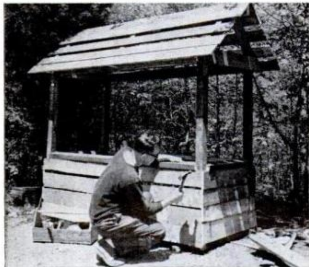
SHEATHING can be any scrap 1-in stock. Random gaps don't matter, since the shingles will cover them
