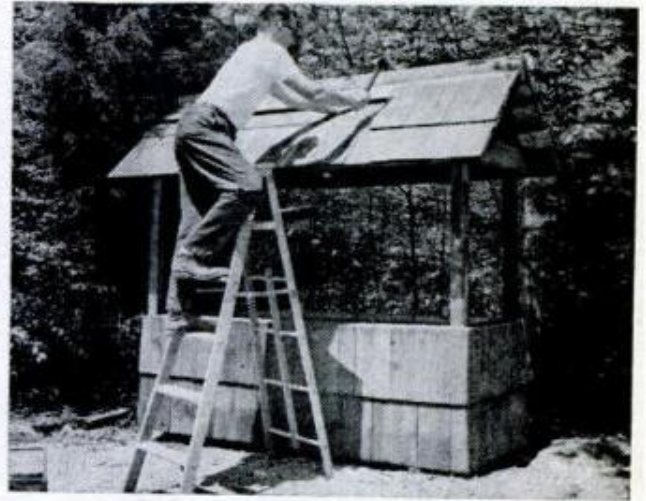
SAME SHINGLES were used on roof, since quantity hardly justified buying a bundle of roofing shingles
