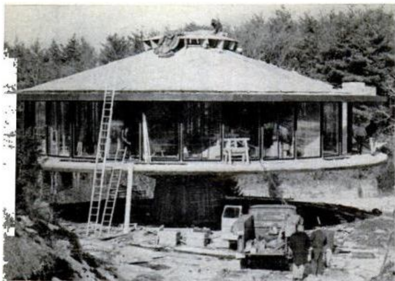
EXCLUSIVE CONSTRUCTION PHOTOS were taken last spring. House will be completed this summer, too late to include photos here. Note that porch guard rails were still to be installed, above. Underbody had been insulated and sheathed with plywood, below, but lacked the shingles
