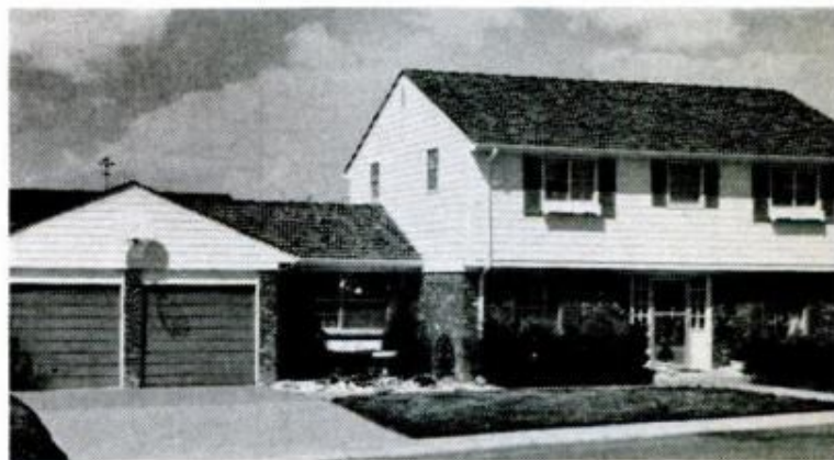
3 YEARS, COLORADO. "Had to paint four times in two years because of severe blistering. Then tried Spred House Paint in 1965. It stopped the blistering and looks great." D. M. Craig.
