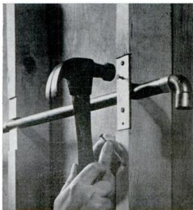
WHEN NOTCHING TUBING INTO STUDS, nail short lengths of strap iron over tubes and flush with studs to keep from puncturing tubes when paneling room
