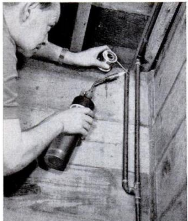
AIR CHAMBERS TO CUSHION SHOCK can be installed as shown at the left, or added as shown above
