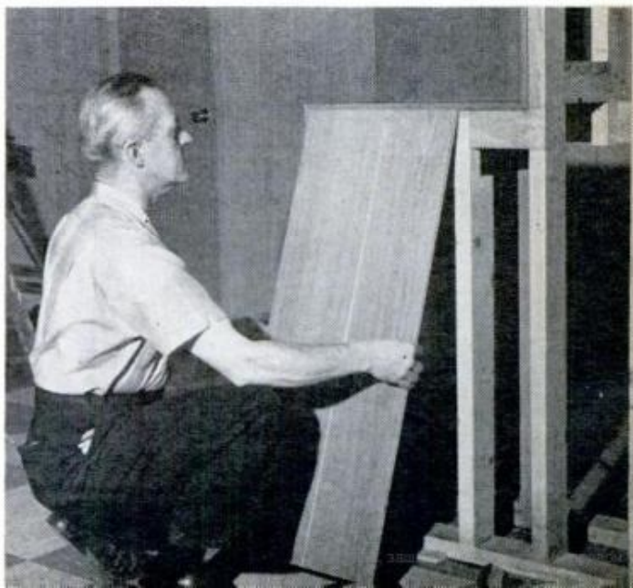
STARTING PANEL is inserted in channels of molding. Work from left to right; leave 1/4-in. space at floor
