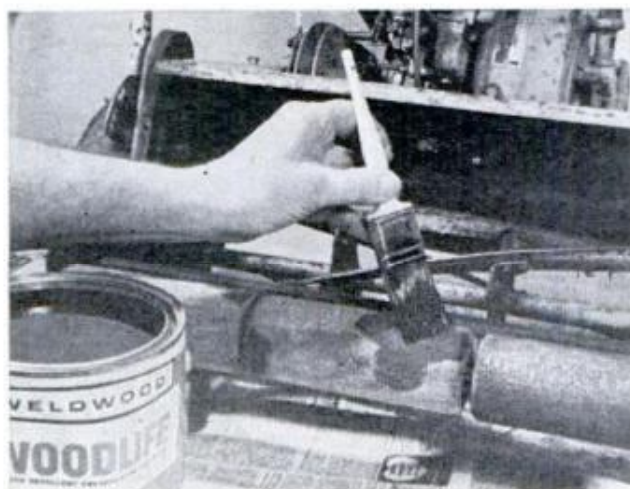
PROTECT WOOD ROLLER on a reel mower by treating it with as much wood preservative as it will absorb
