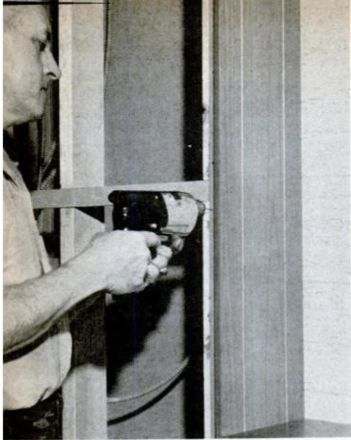
FLANGE OF MOLDING is first drilled every 4 in. for 1-in. nails that are used to fasten it at corners
