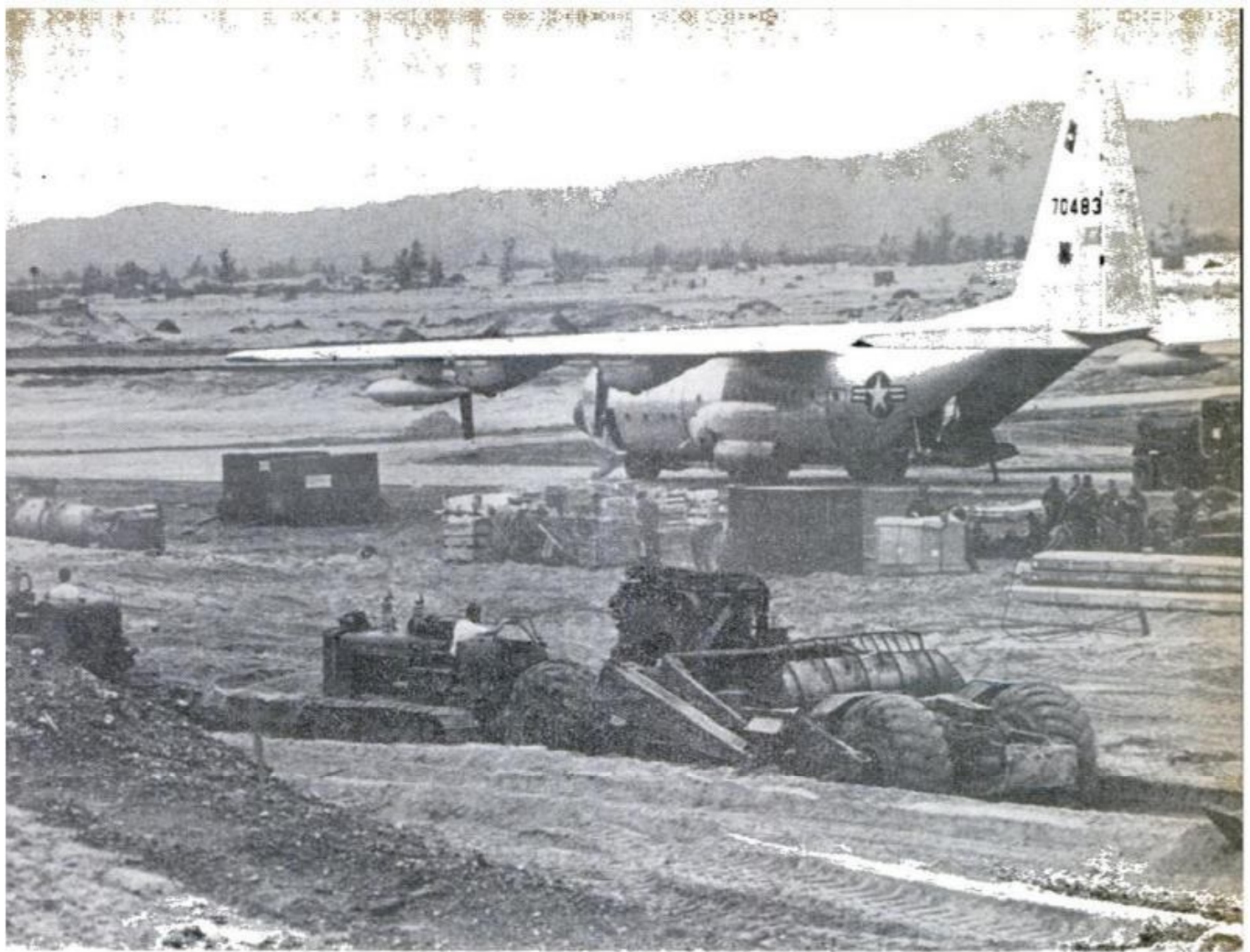
MAJOR WORKLOAD is construction of new airfields. Another is building of whole communities for troops
