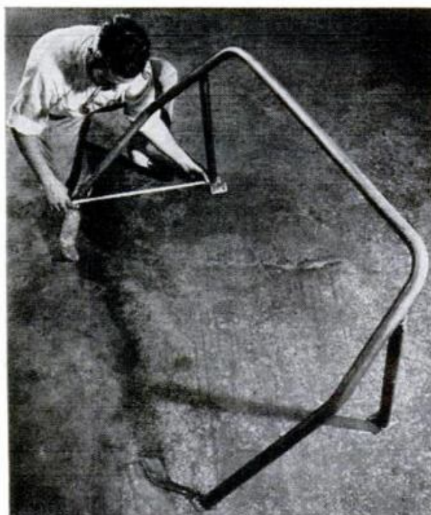
CHECK ALIGNMENT of braces—difference should be only a fraction of an inch. Then complete all welding
