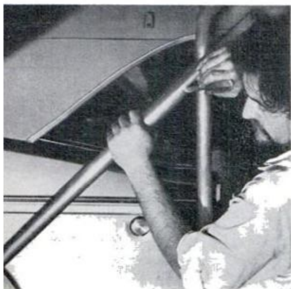
BRACE TUBING is fitted and marked, and then cut to approximate required length
