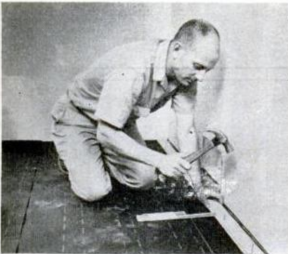
FIRST COURSE is aligned and face-nailed in place
