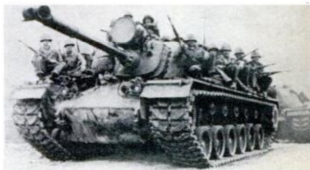
TIME OUT for Seabees from building job often means combat duty, trading picks and shovels for guns
