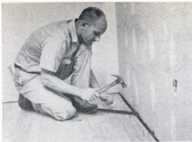
LAST COURSE also is face-nailed. Bar tightens fit
