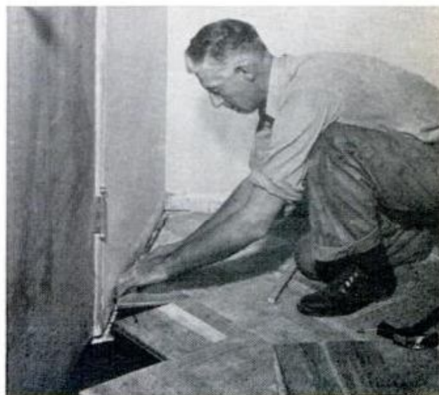
BLOCK FLOORING is commonly laid on asphalt mastic
