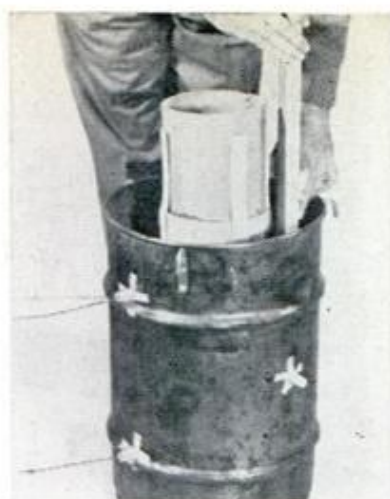
CORE IS PLACED in drum with 4-in. Firecrete bottom, then cast
