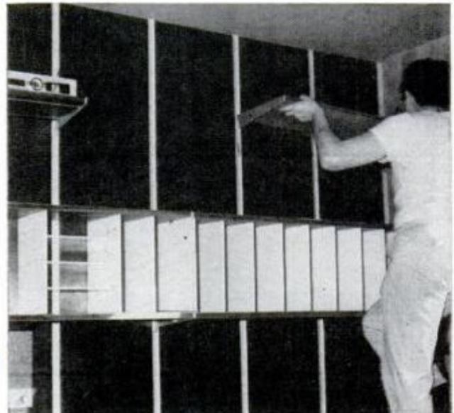
LOCKING BRACKETS in tracks support ready-made shelves and cabinets in any grouping desired
