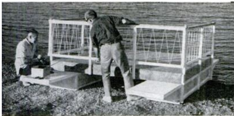
BOLT DECK PANELS to pontoons, then secure both front and rear rail to deck panels and the side rails
