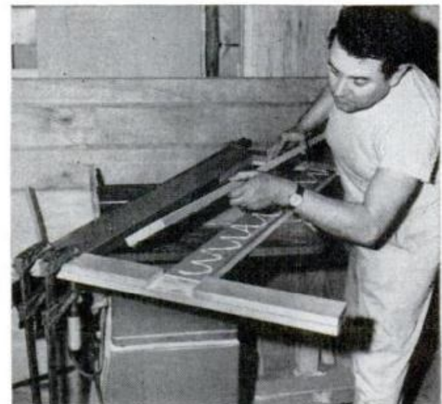
TRAIN-BOARD LEGS and crossrail can be 2x4s or built up of two 3/4-in. pieces and glued in dadoes
