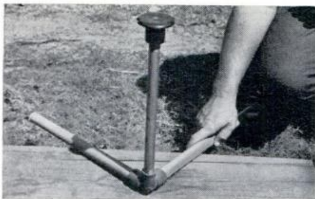
PUT OUTLETS in corners by using 3-way fitting with top threaded socket, slip fittings at bottom
