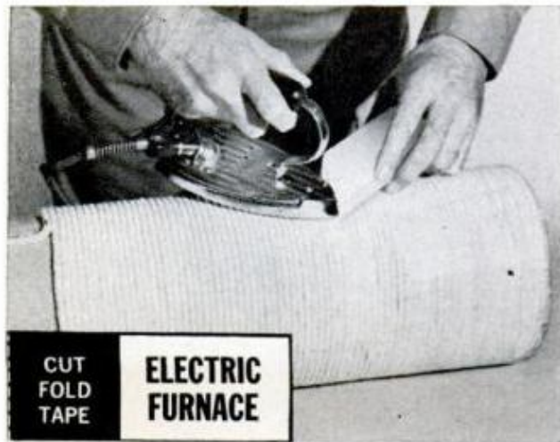
HEATED PARAFFIN is forced between ridges of cord. This will provide a smooth surface inside refractory
