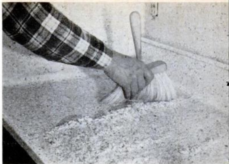
EXCESS FLAKES can be brushed up once base coat has set. Save these for next section to be covered
