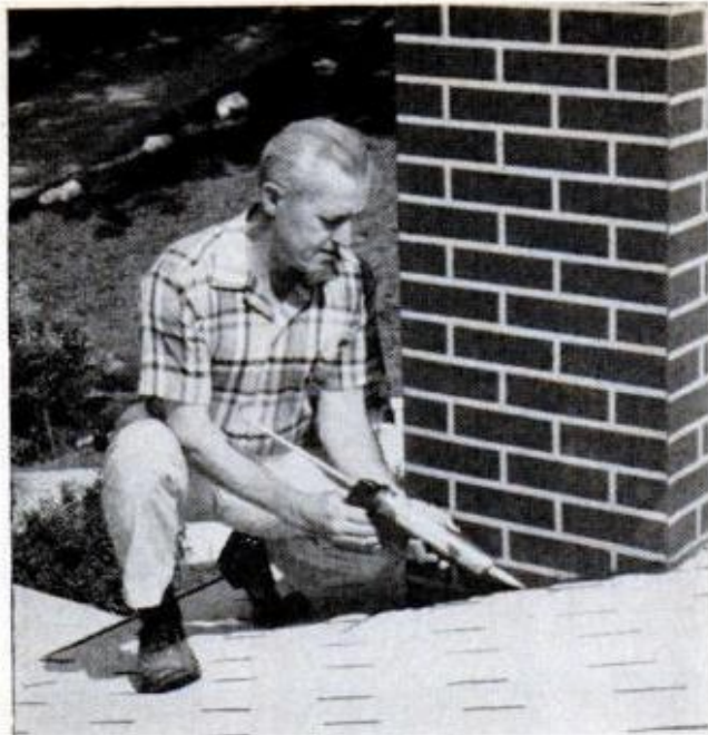
CAULKING IS APPLIED to shingles and flashing to make the chimney housing watertight at the roof line
