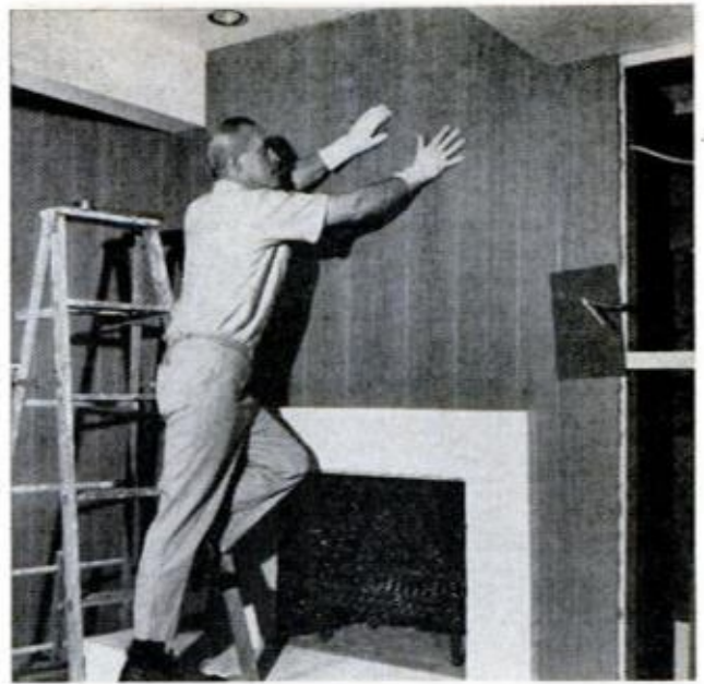
RUBBER GLOVES afford a nonslip grip in forcing slick-finish paneling in place. Avoid tight tongue-and-groove joints. Leave \frac{1}{16} -in. space for expansion
