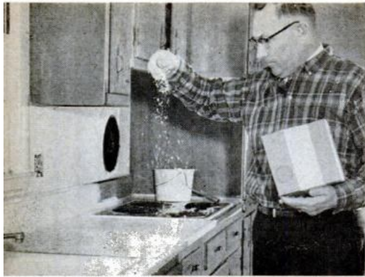
TOSS VINYL CHIPS so they cover the wet base coat. It's best to work only a small section at a time
