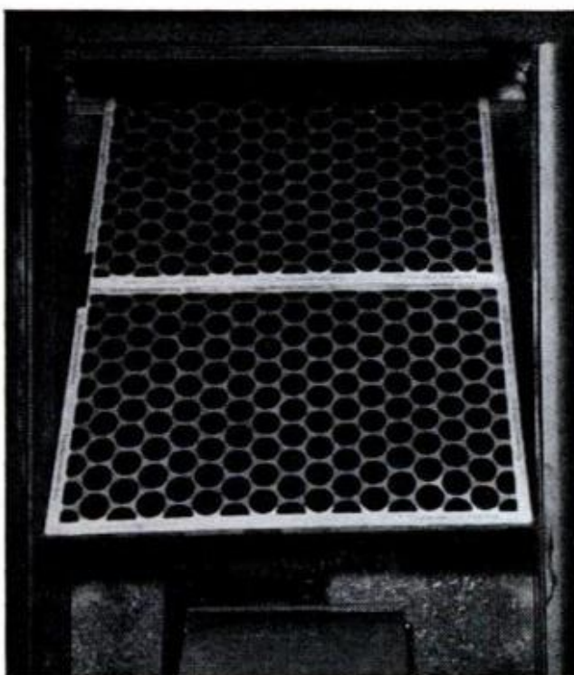
FILTERS in forced-air systems will greatly reduce available heat if dirty or clogged. Check them often
