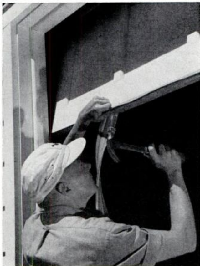
GARAGE-DOOR BOTTOM nailed along the lower edge of door not only plugs leaks but acts as cushion
