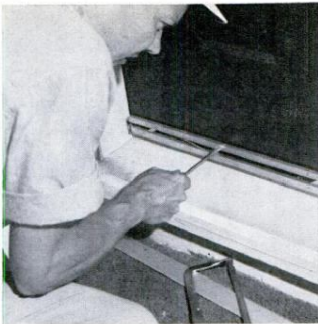
AUTOMATIC DOOR BOTTOM raises when door is open to provide clearance between door and rug
