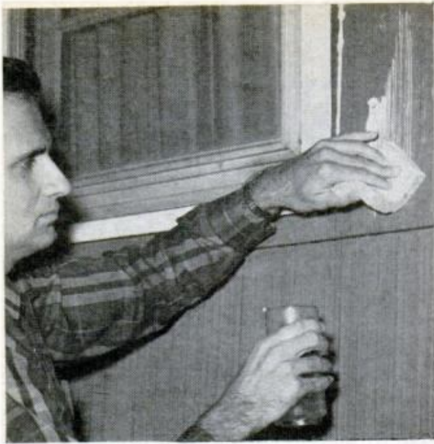
ONE ADVANTAGE of latex caulk is ease of removal before it's fully cured. Plenty of water does the job
