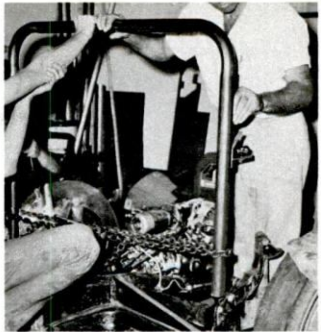
INSTALLING ROLL BAR is two-man job. When level, the bar must be securely welded to the torsion tubes
