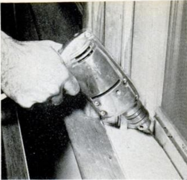
EACH WINDOW should have at least three weep holes to let trapped water escape outside the frame
