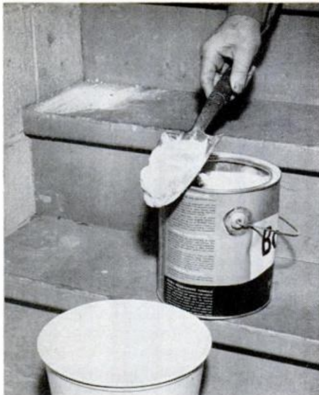
PORTLAND-CEMENT PAINT is sold in powder form. You must mix it with water before you can go to work
