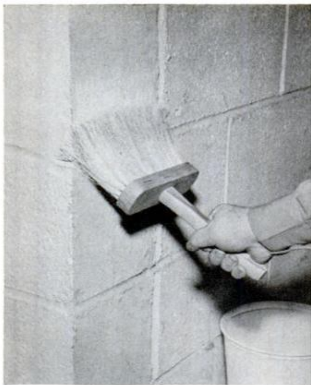
CLEAN SURFACE thoroughly with a wire brush before applying fresh paint to previously finished masonry
