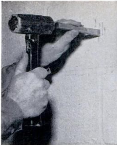
◀ HOLE FOR EXHAUST PIPE is cut through masonry wall with cold chisel. Caulking seals the tubing
