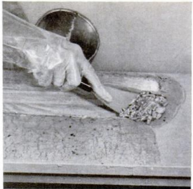
THICK, GOOEY SLUDGE , left after paint remover has softened and loosened the old finish, must be scraped off. Best tool for this is a broad-bladed putty knife. Be sure to wear gloves at all times
