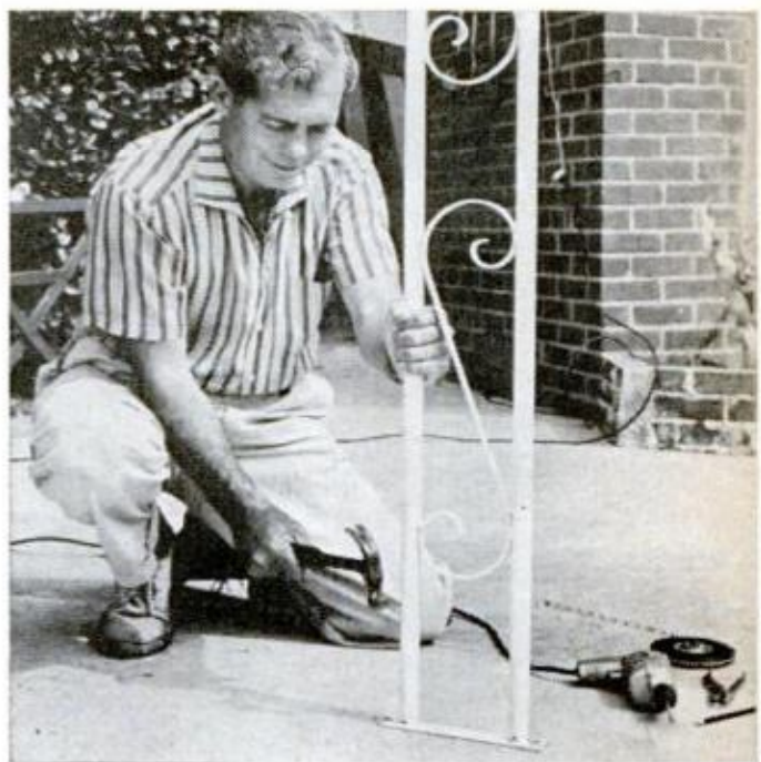
ORNAMENTAL POSTS have mounting flanges on both ends, are secured to concrete by driving tampons into predrilled holes. Use star drill or masonry bit for this
