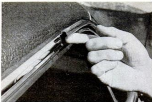
SPECIFIC WORKMANSHIP COMPLAINTS included loose chrome and molding fit; example is rain gutter
