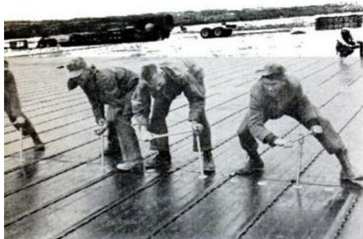
MATTING PALLETS are mated together, then bolted into place at overseas base. Smooth surface leaves only catapult dolly and arresting cables above ground
