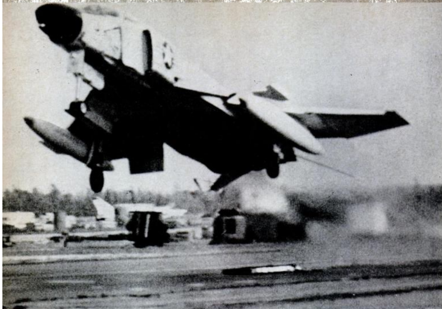
F-4 PHANTOM roars off short airfield, outrunning catapult dolly. Dolly slides over shallow groove in matting where "Chinese fingers" grab firm hold on continuous cable. It can throw aircraft into air in much less than 2200 feet required for SATS airfields. Pilot keeps stick "full aft" for quick getaway
