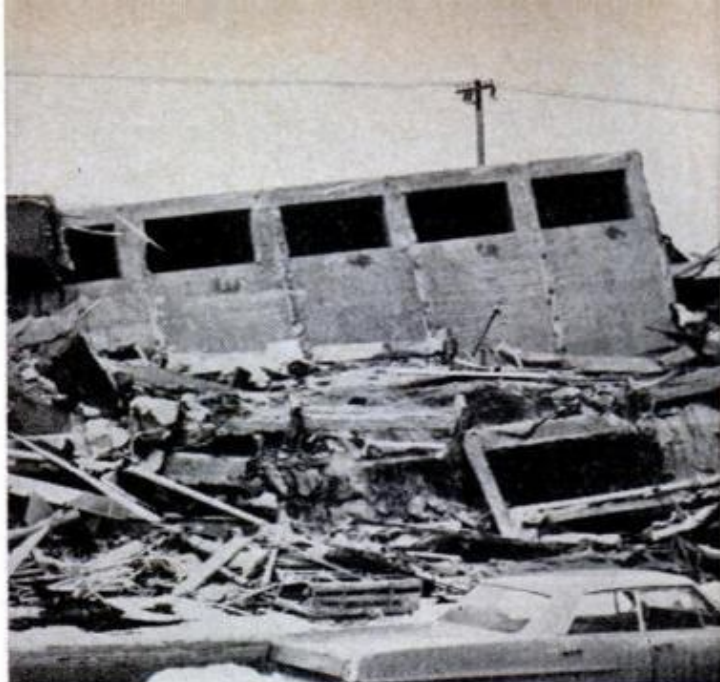
PILE OF RUBBLE above was all that remained of six-story apartment building in Anchorage, Alaska, after '64 quake. Connections between floors and columns gave way, collapsing the whole structure. Below, hydraulic jacks simulate earthquake stress on an actual-size test frame at Lehigh University
