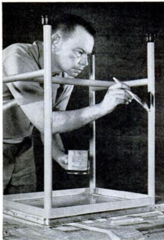
FOR LASTING FINISH , prime welded pipework with a rust-inhibiting primer, then brush on at least two coats of any good-quality, synthetic-base enamel
