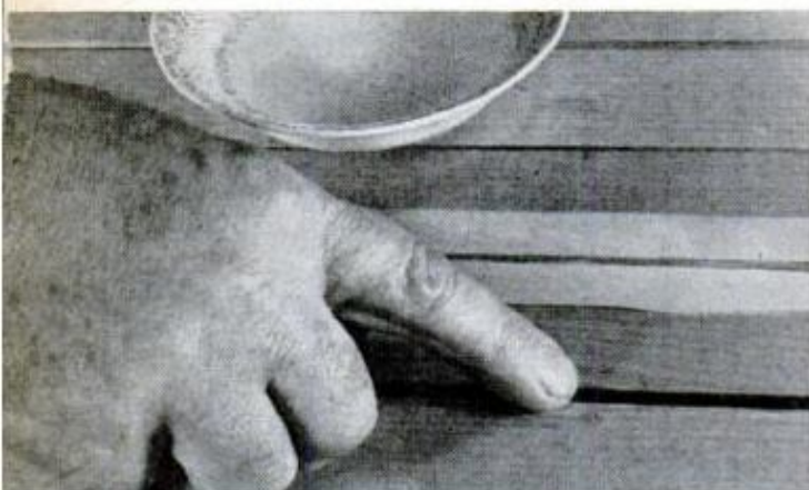
YOUR MOIST FINGER is best tool for smoothing a polysulphide seam to proper concave configuration
