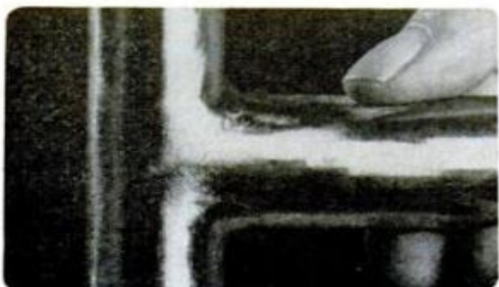
4. SAND JOINT to remove remaining scale
