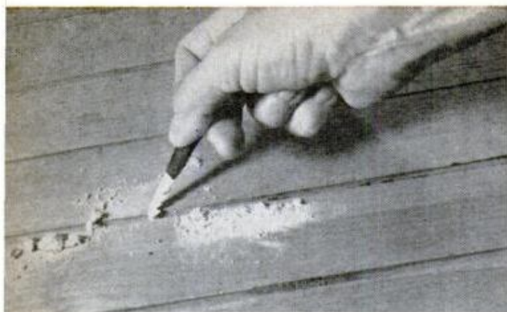
MAKE THIS TOOL for cleaning seams by wrapping tape around broken sabre-saw blade to form handle
