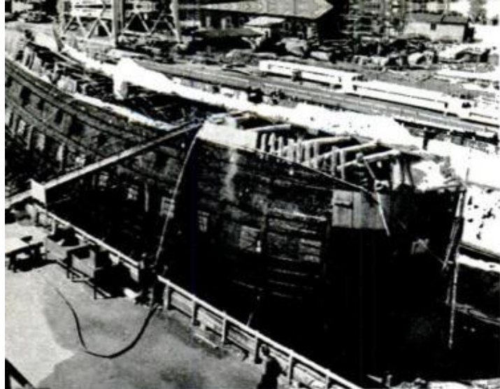
WASA FLOATED INTO DRYDOCK 10 days after she was first brought to the surface. Now she rests under a roof on a specially built concrete pontoon
